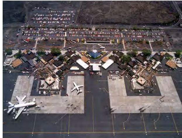
Various Construction Projects, Kona International Airport (1998-2009)
