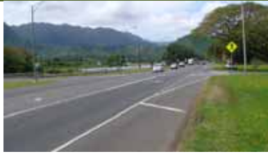
Kahekili Northbound Approach at Ahaolelo
