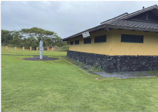
Existing comfort station at Isaac Hale Beach Park
