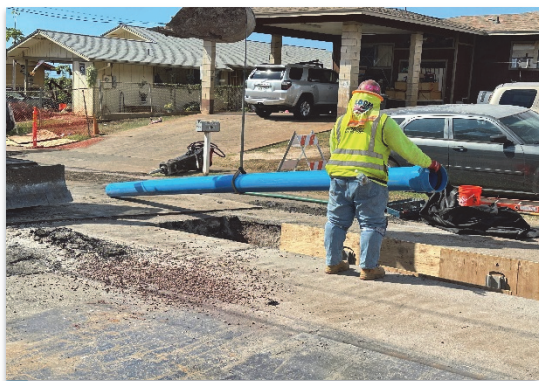
Sewer line replacement in Wai'anae
