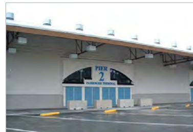
Pier 2 Cruise Terminal, Honolulu Harbor, Oahu (2006)
