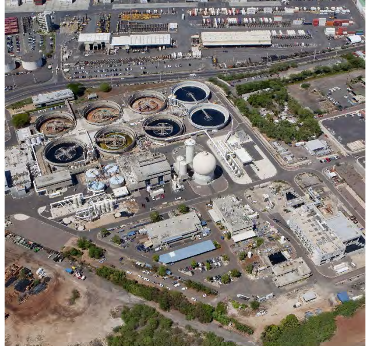
The Sand Island 90-mgd Wastewater Treatment Plant (WWTP) is the State of Hawaii's largest, serving metropolitan Honolulu. Beginning in 2006, RMTC provided the design for two upgrade and modernization projects totaling over $70 million in construction cost.
