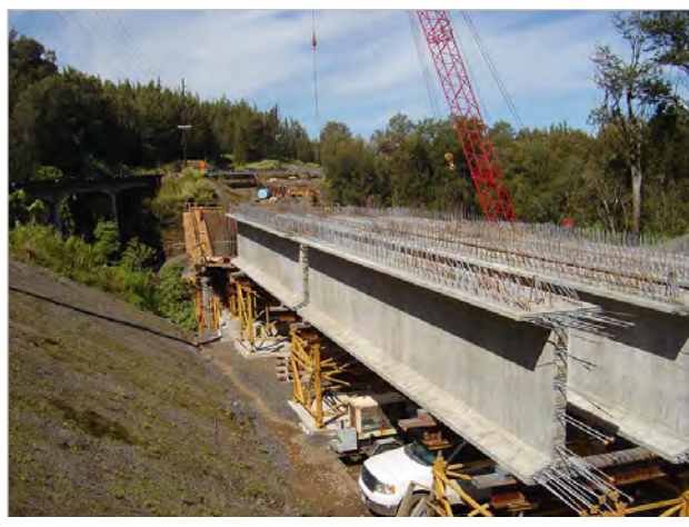
Kealakaha Stream Bridge Replacement, Hawaii (2010) Construction Cost: $36M
