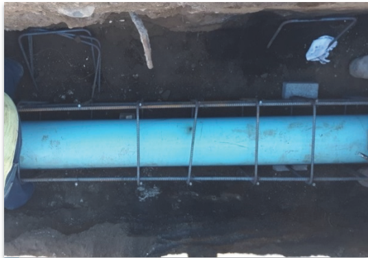
Installation of new 8-inch sewer line within the intersection of Punchbowl Street and Queen Street
