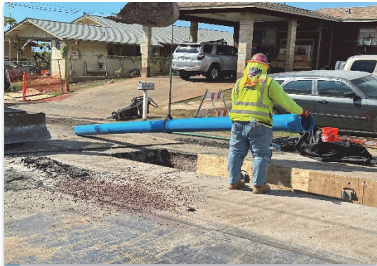
Sewer line replacement in Wai'anae
