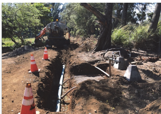
New 4-inch irrigation water line pipe and lateral installation in the Lower Hamakua Ditch Watershed
