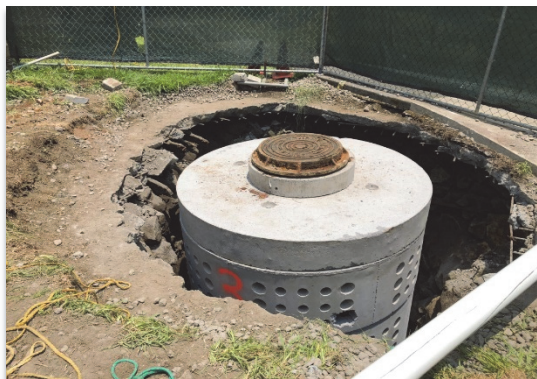
Seepage pit installation at Nani Olu
