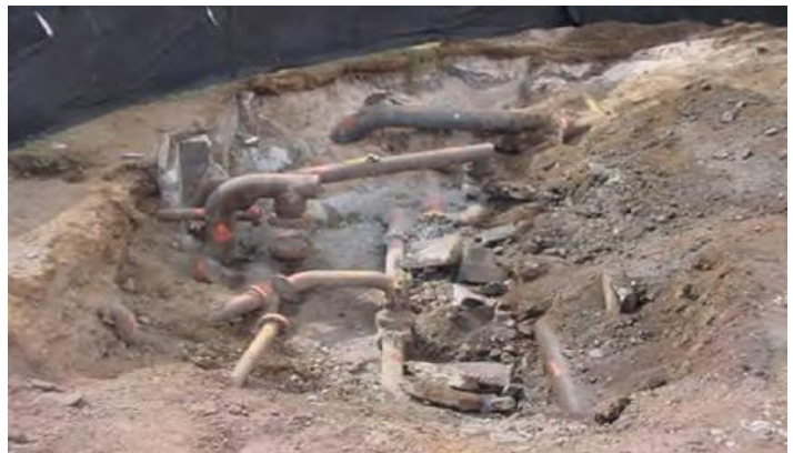
Buried fuel pipelines evaluated near Honolulu Harbor
