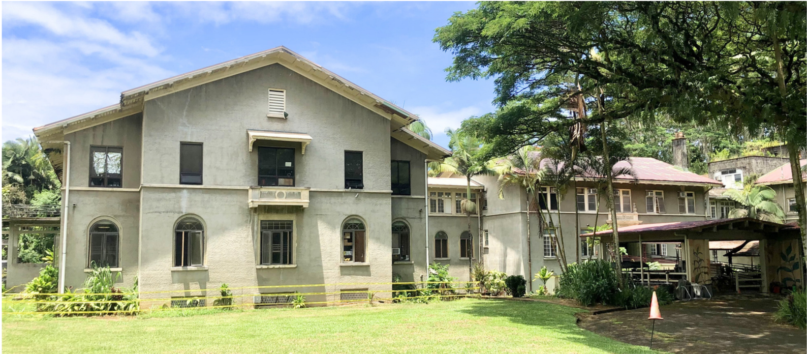
Hilo Memorial Hospital, which is set to undergo renovation starting this year, is seen in this August 2025 photo. County of Hawai'i photo
