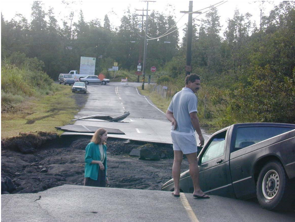
Figure 4 - 22 Damaged Road Surface at Kuauli Road
