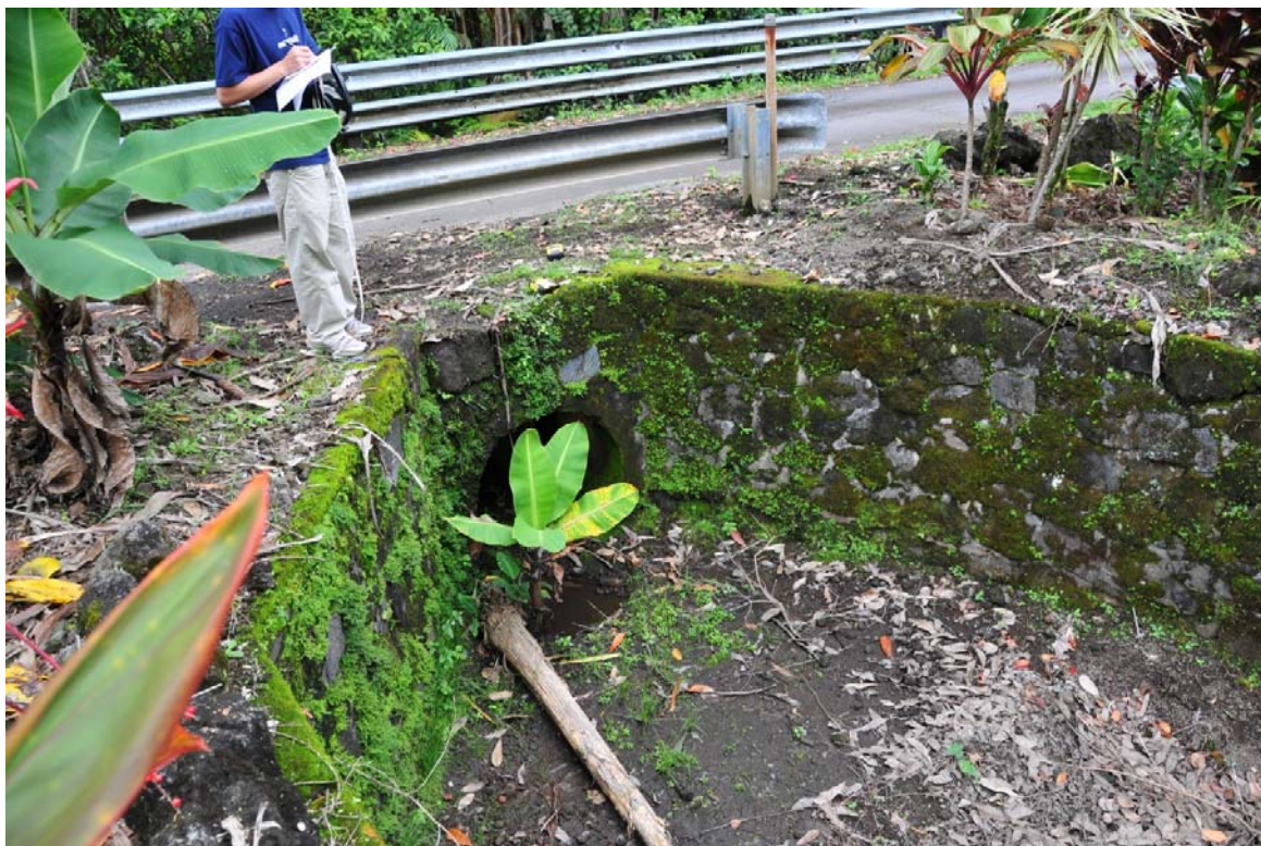
Figure C- 18. Photo of Enos Road Culvert.
