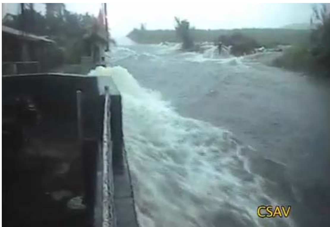
Figure 4 - 20 Flood Waters Flow over the Kukui Camp Road
