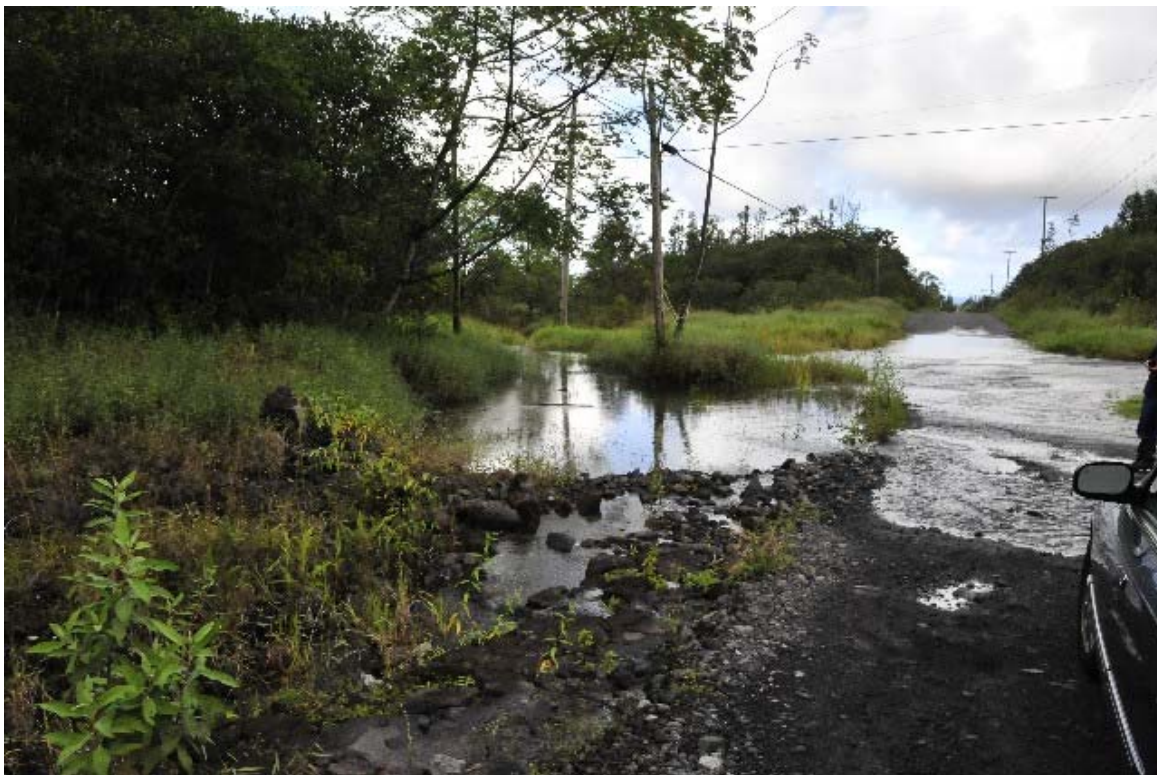
Figure 4 - 7 The Intersection between the 39th Avenue and Pohaku Drive
