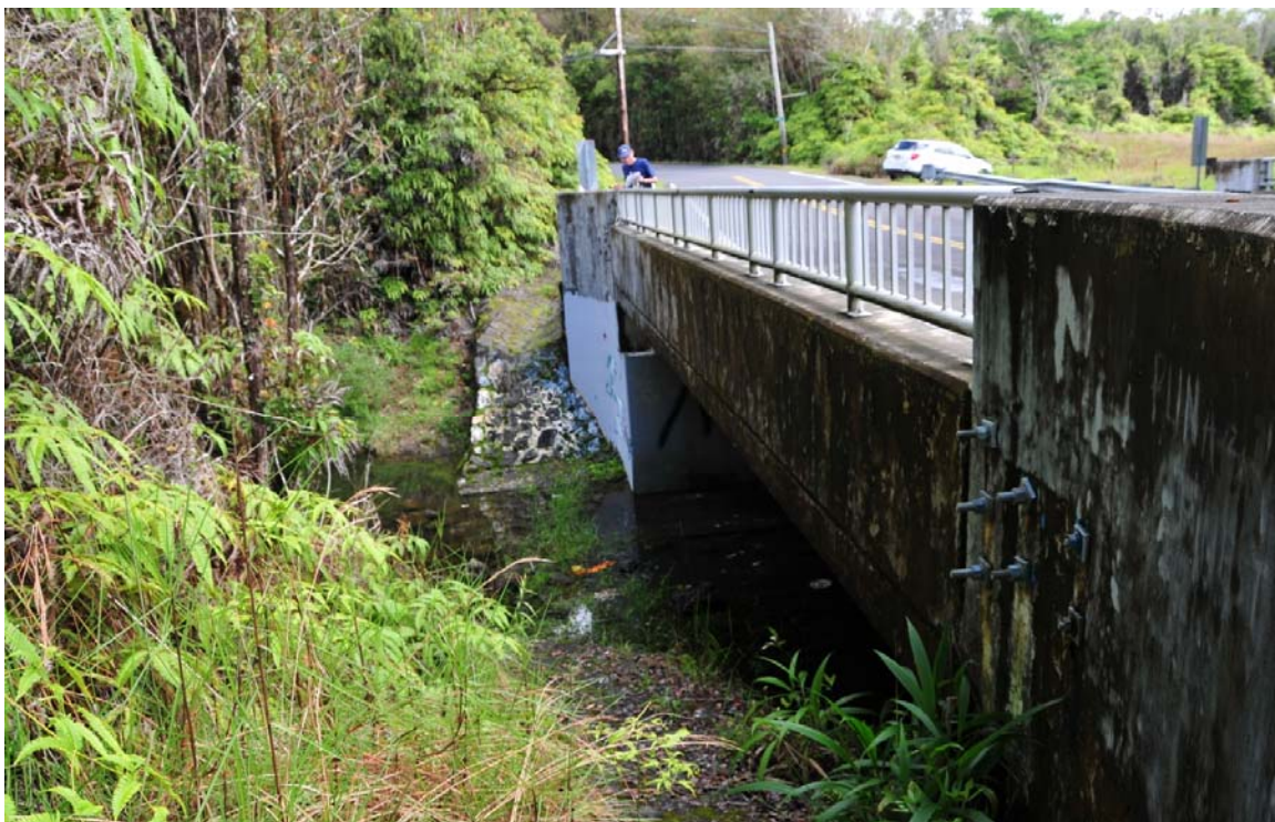
Figure C- 30. Photo of North Oshiro Road Bridge 2.
