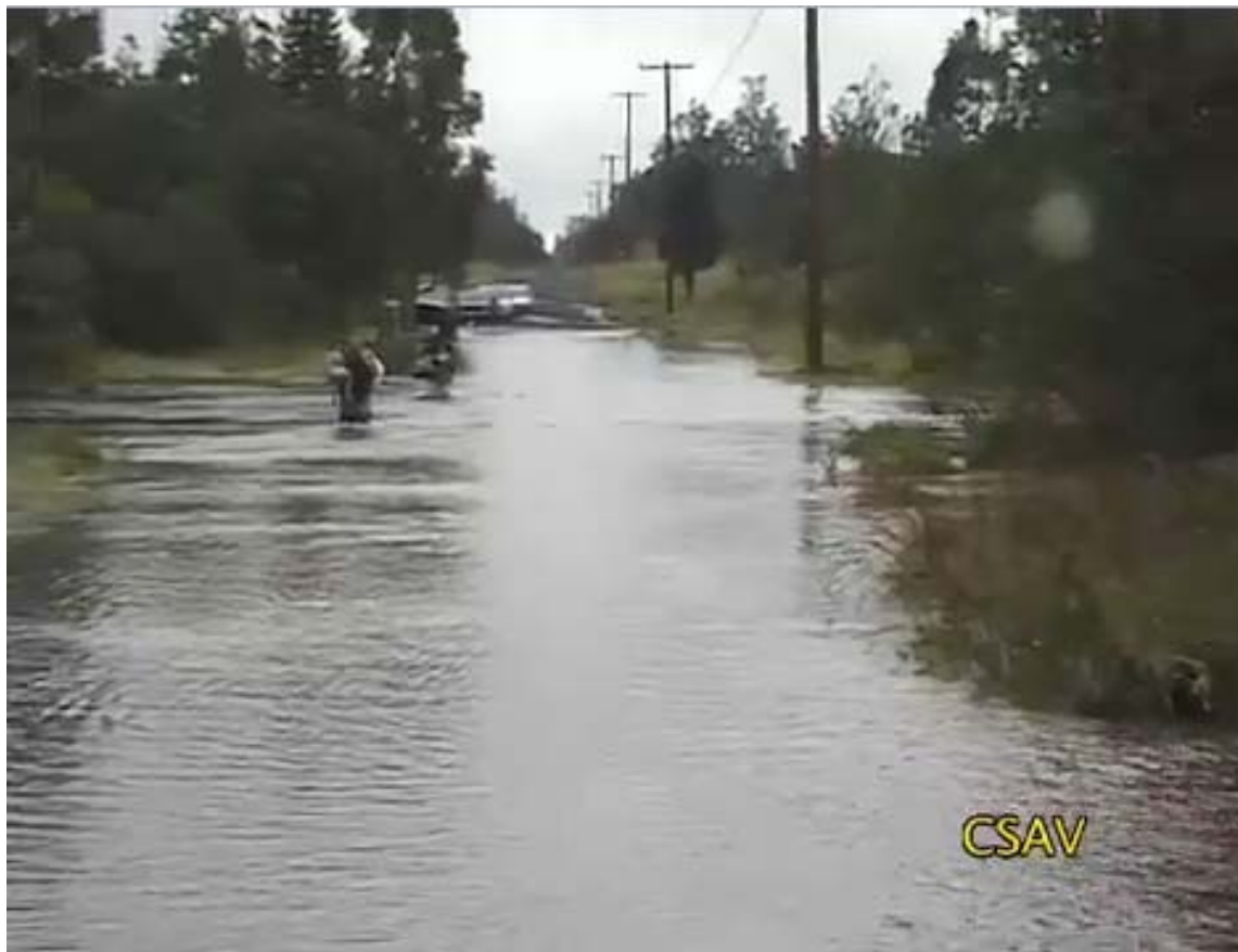
Figure 4 - 18 Flooded Roads at Puna District
