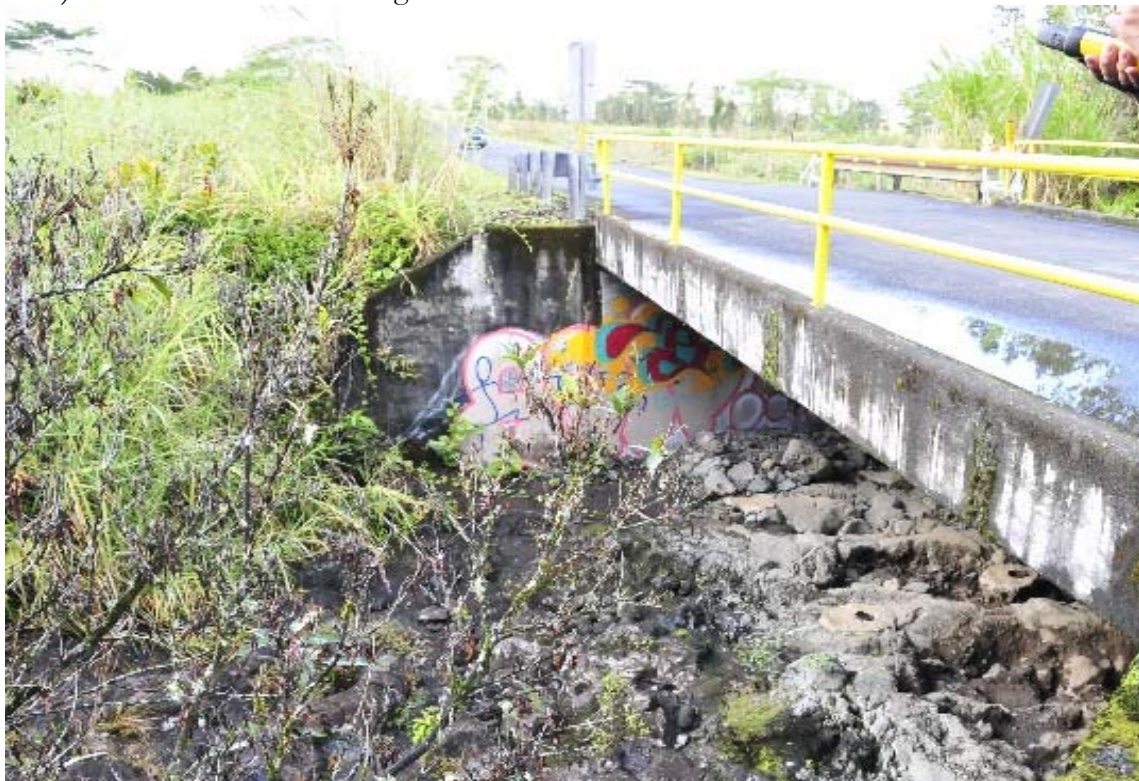
Figure C- 15. Photo of South Kūlani Road Bridge.
