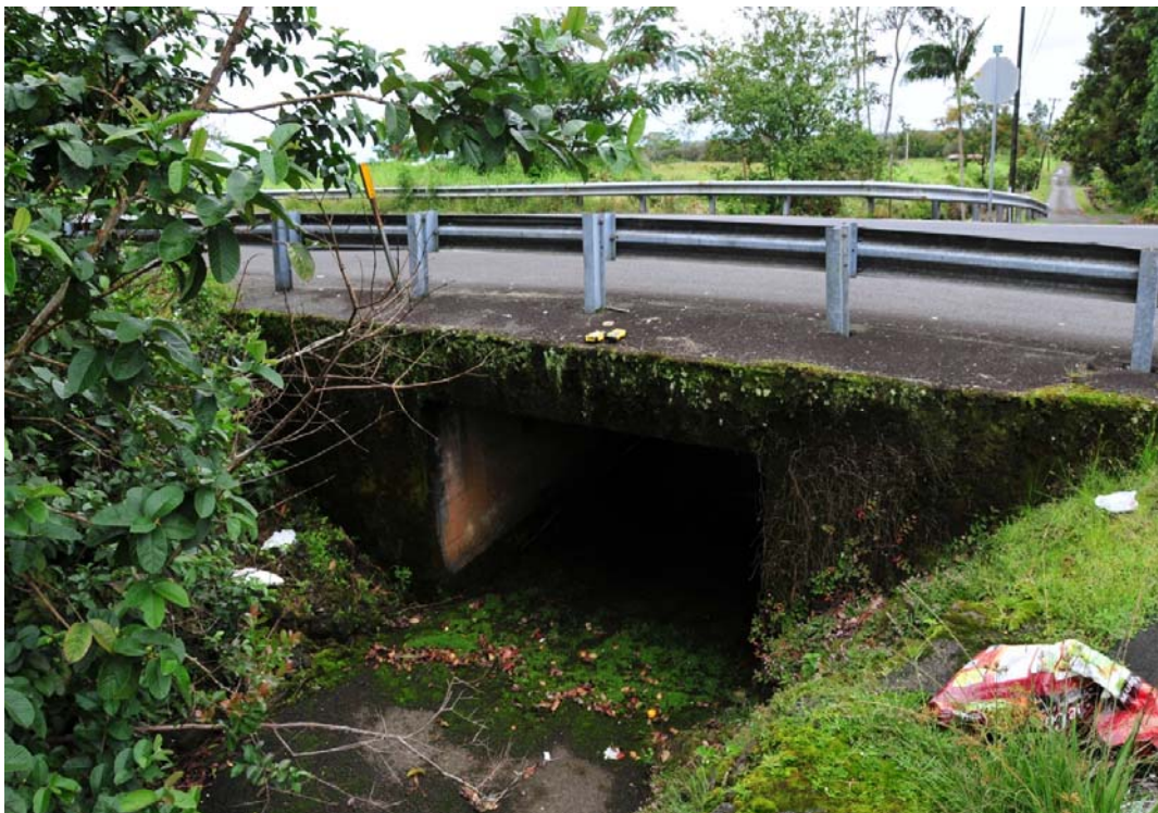
Figure C- 23. Photo of South Pszyk Road Culvert 2.
