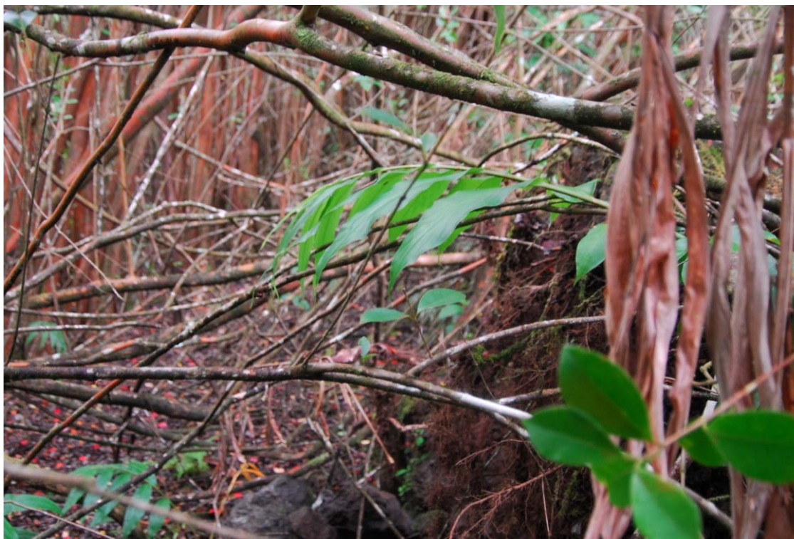
Figure 4 - 13 Failed Section of Rock Wall
