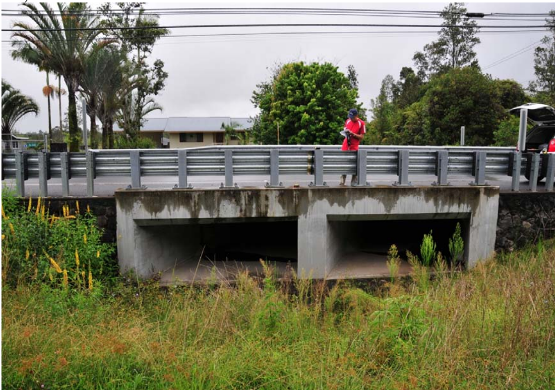
Figure C- 9. Photo of Moho Road Culvert 1.
