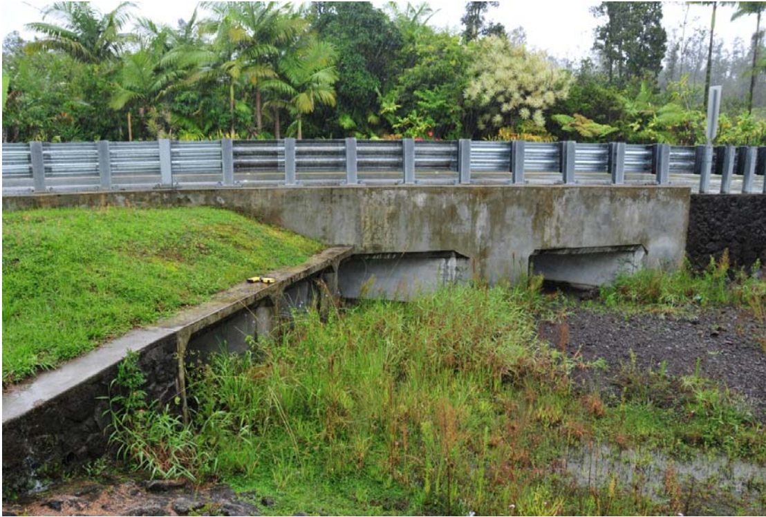
Figure C- 12. Photo of Moho Road Culvert 2 (Downstream side).
