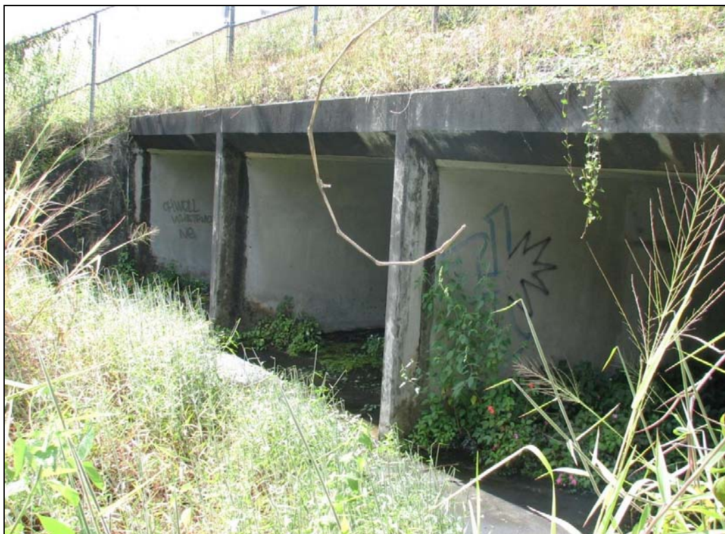
Figure C- 2. Photo of the Keaau-Pahoa Road Culvert 1.
