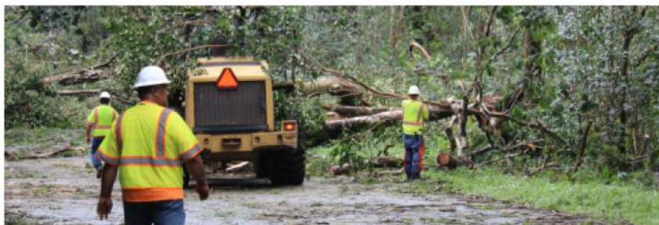
A county work crew removes albizia trees.
