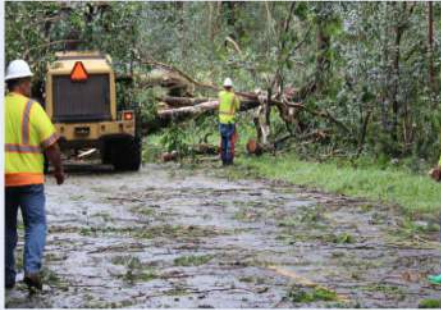
County crew clearing albizia trees.
