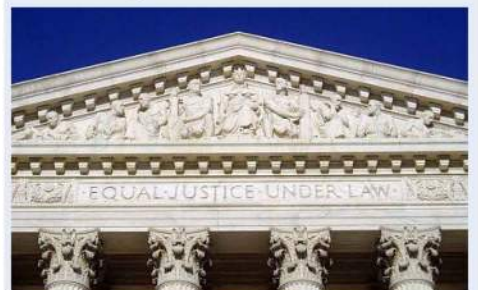
"Equal justice under law" is engraved on the facade of the Supreme Court building
