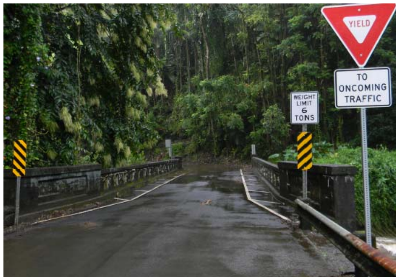
Insert 2. Looking south from north abutment.
