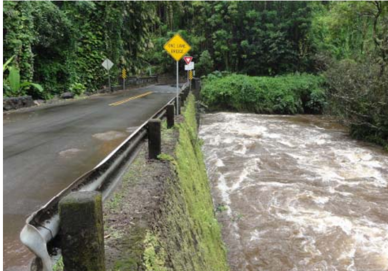
Insert 3. View of “Rock Embankment” north of north abutment, looking south.
