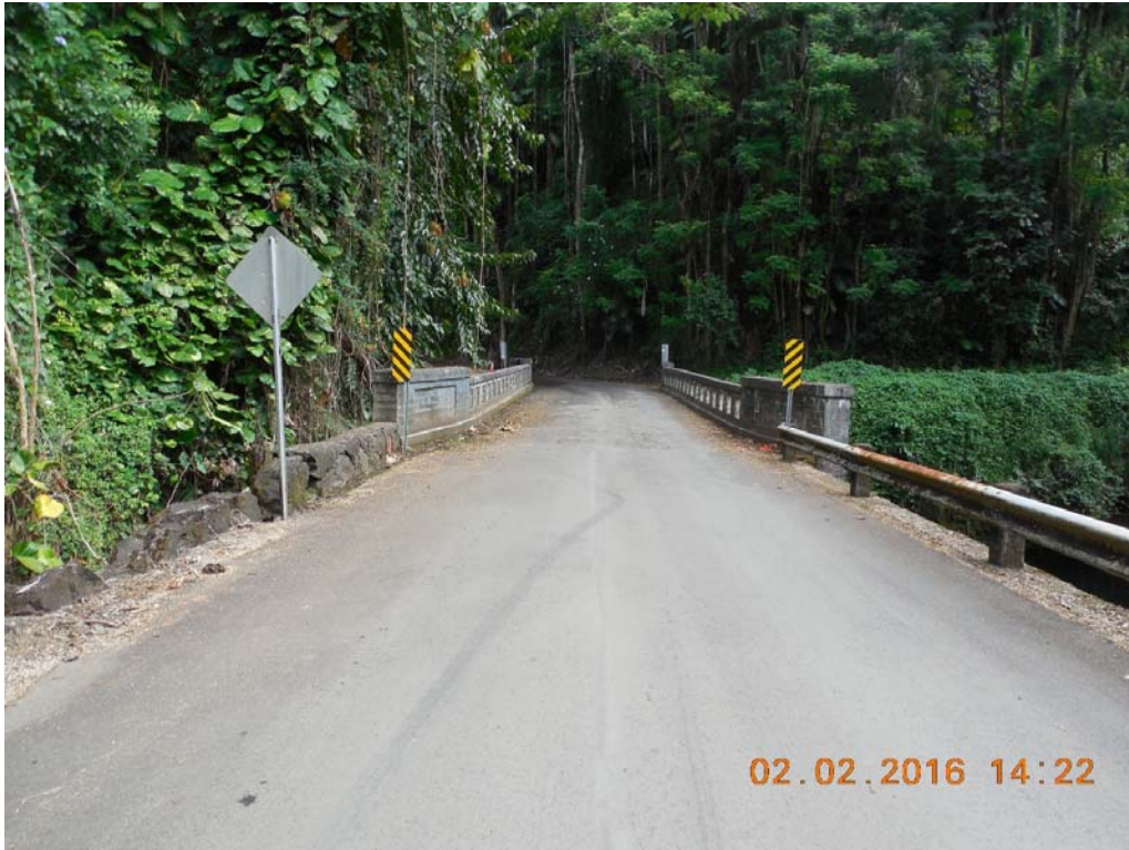
B1: View of the Hakalau Bridge from the roadway from north approach.
