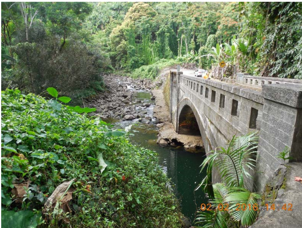
B2: Upstream bridge profile.
