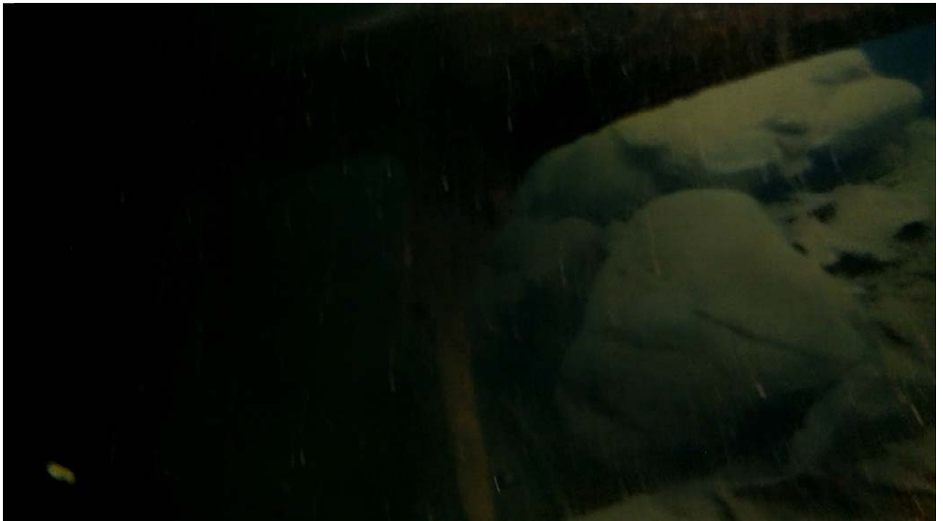
B17: SOUTH ABUTMENT (UNDERWATER) Underwater photo below the rock of the upstream side (Refer to photo B7).
