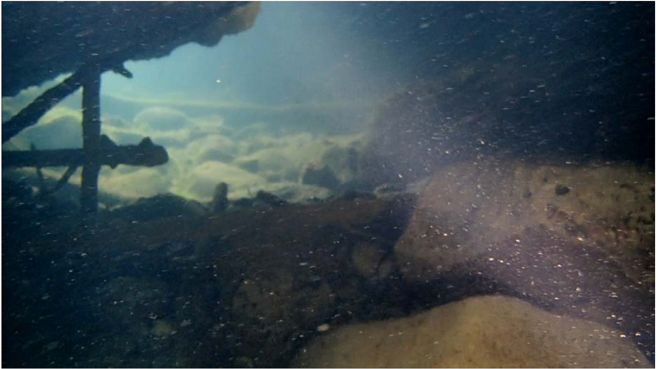
B21: NORTH ABUTMENT (UNDERWATER) Near downstream-side entrance.
