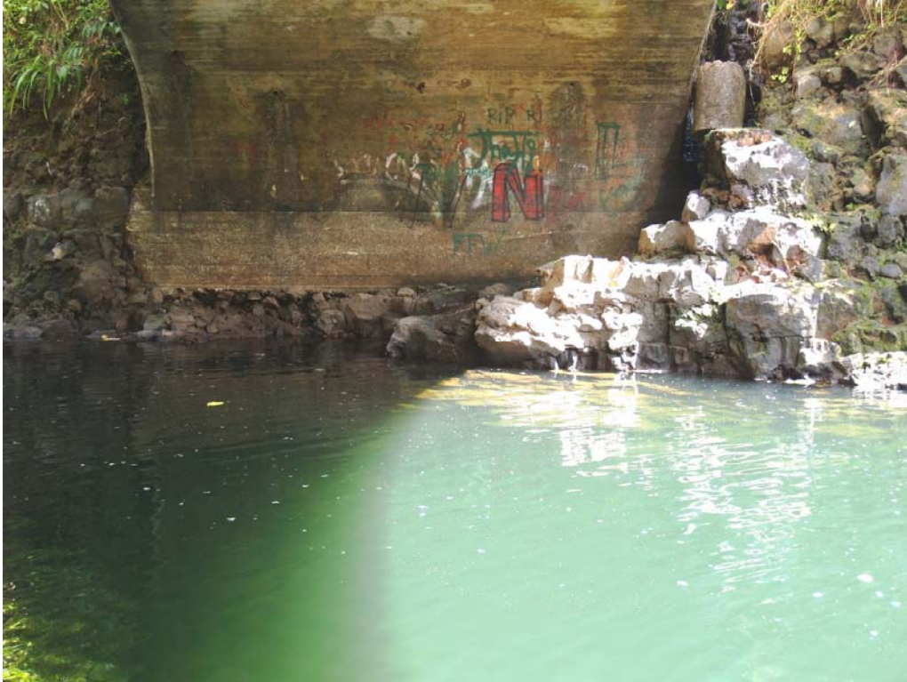
B7: South end abutment & rock ledger.
