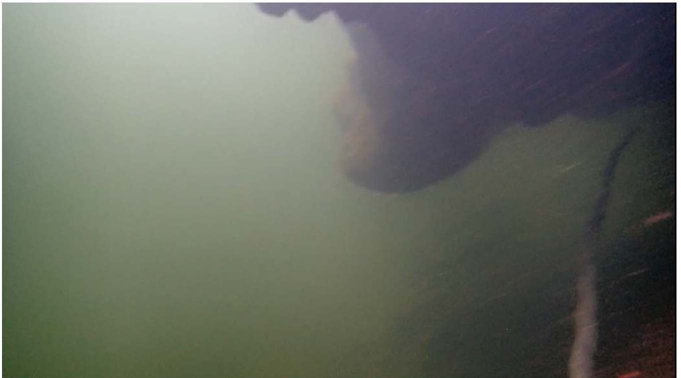
B18: NORTH ABUTMENT (UNDERWATER) Upstream entrance.
