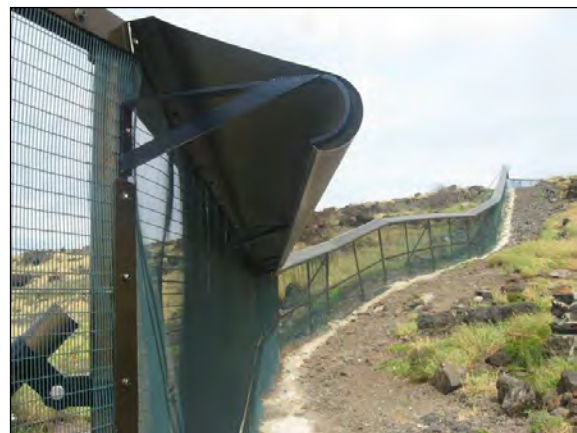
PREDATOR FENCE AT KA'ENA POINT, O'AHU
