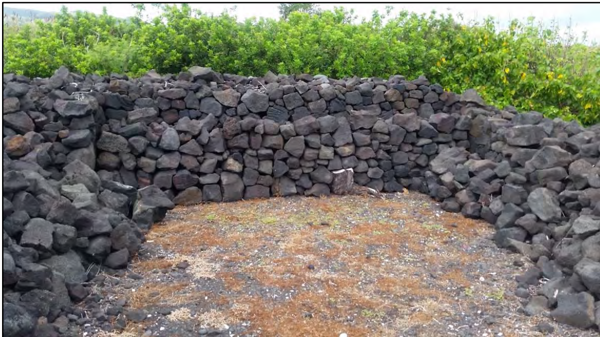
INVASIVE VEGETATION REMOVED NEAR A HOUSE SITE
