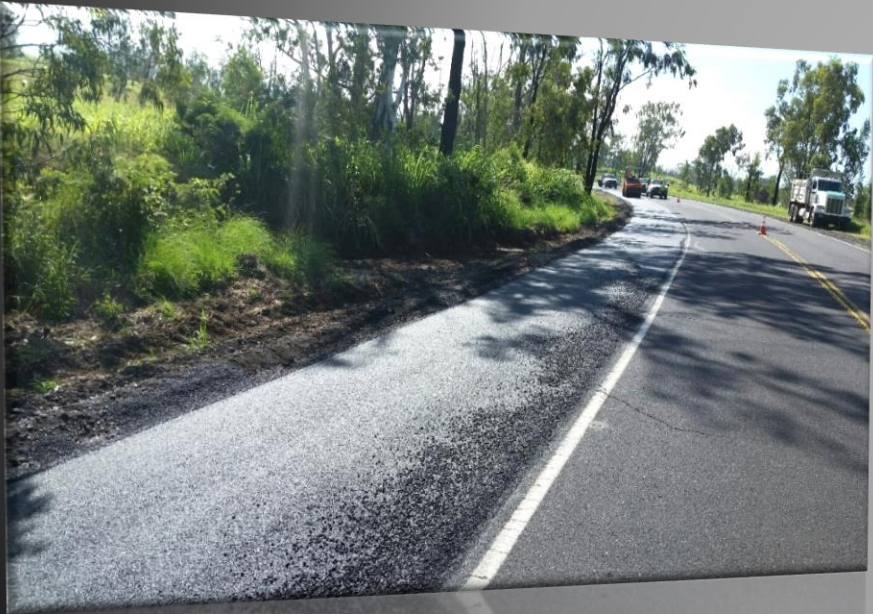
The construction of nine foot asphalt concrete shoulders on both sides of the Waikoloa Road, from Highway 190 to Queen Ka'ahumanu Highway.
