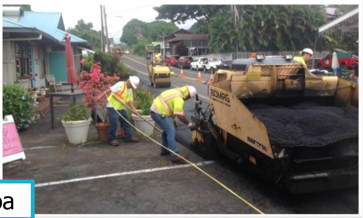
The construction of nine foot asphalt concrete shoulders on both sides of the Waikoloa Road, from Highway 190 to Queen Ka'ahumanu Highway.
