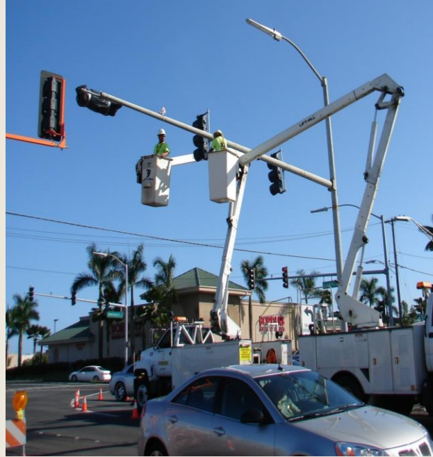
Traffic Signal Maintenance, S. Hilo
