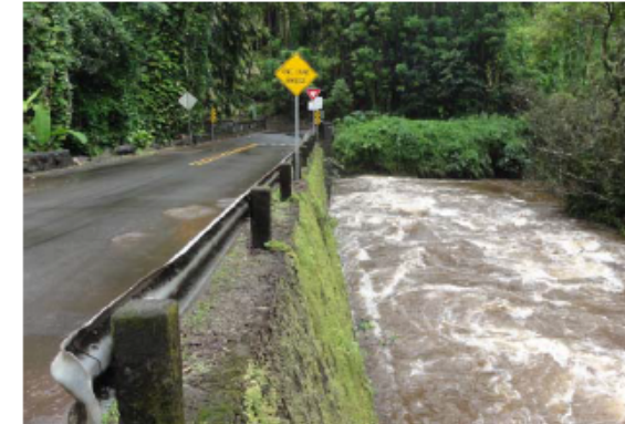
Insert 3. View of “Rock Embankment” north of north abutment, looking south.
