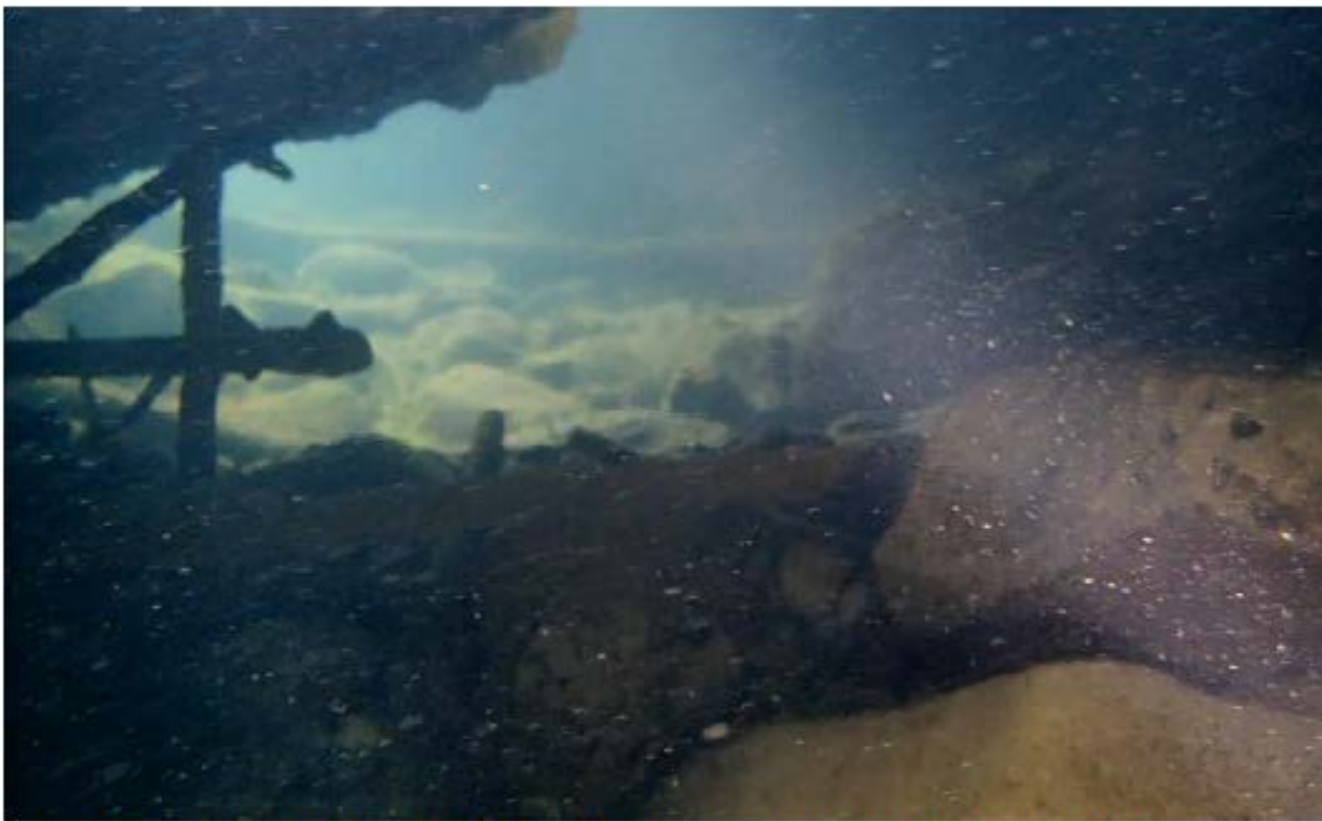
B21: NORTH ABUTMENT (UNDERWATER) Near downstream-side entrance.
