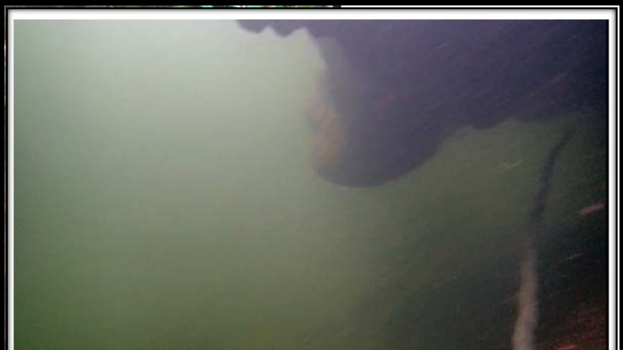
B18: NORTH ABUTMENT (UNDERWATER) Upstream entrance.
