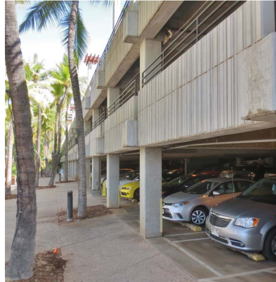
Parking garage at Fort DeRussy in Waikīkī.
