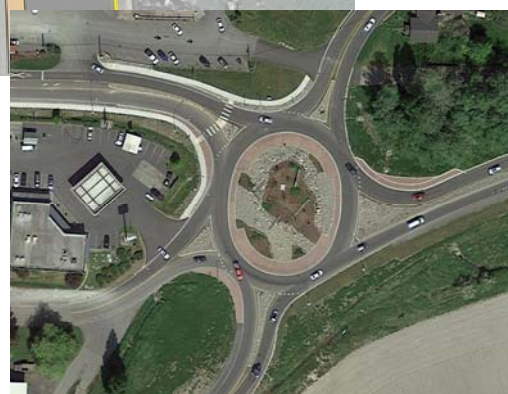
Inset: 5-leg roundabout, Pioneer Hwy, WA
