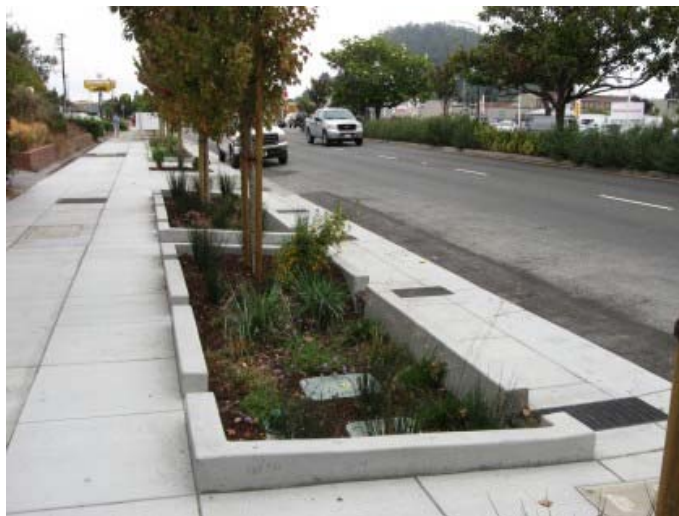
Example of an urban Green Street design using a continuous bioswale planter with drain inlets along the sidewalk and parking lane. (Portland, OR).
