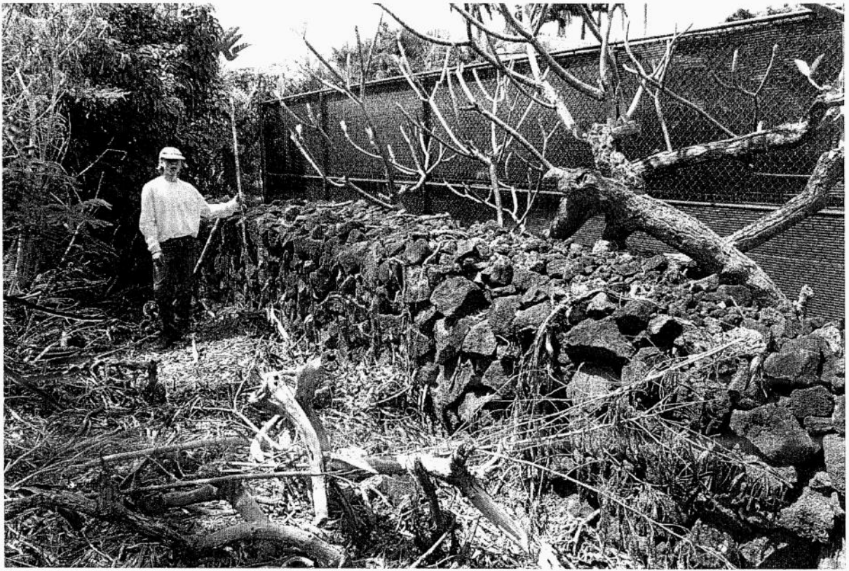
Photo 5 Intact portion of core-filled wall.
