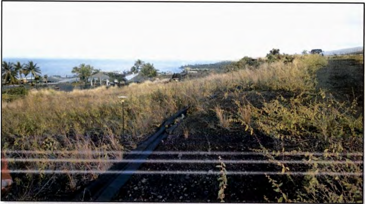
Figure 4. Overview of project area showing bulldozed cut and silt fence, view to northwest
