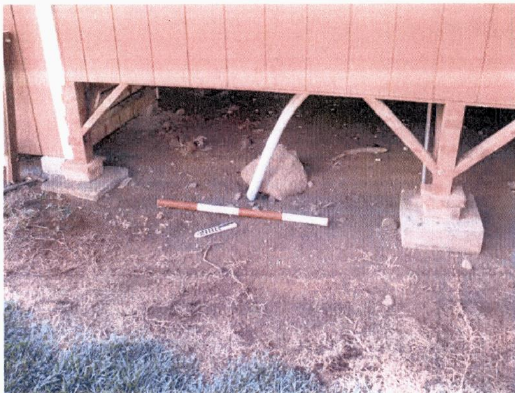
Figure 4. Inadvertent discovery area under corner of building, view to the southeast.
