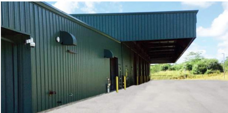
Figure 5-1. Hilo Baseyard Facility
