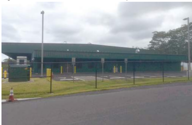
Figure i-4. New Transit Maintenance Facility on Hololaulima Road
