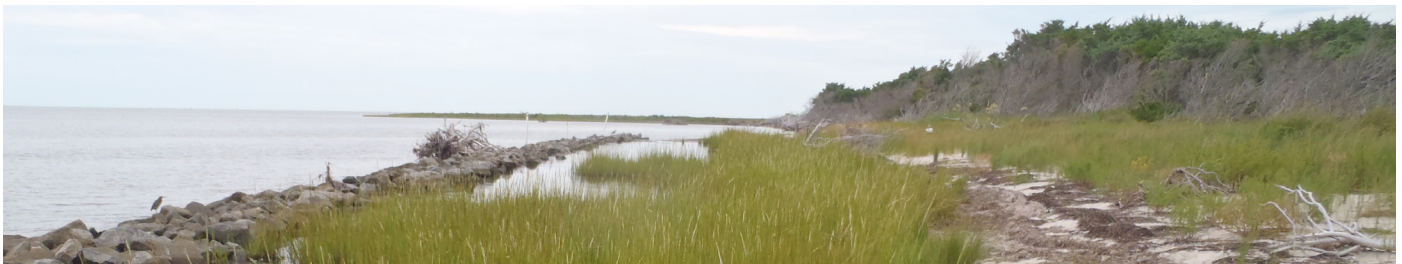
Hatteras, NC. The Durant's Point living shoreline project protects the shoreline from storm surge while providing habitat for many species. Since its construction, the project has weathered hurricanes, a summer of drought, and tropical storms. Photo: N.C. Coastal Federation
