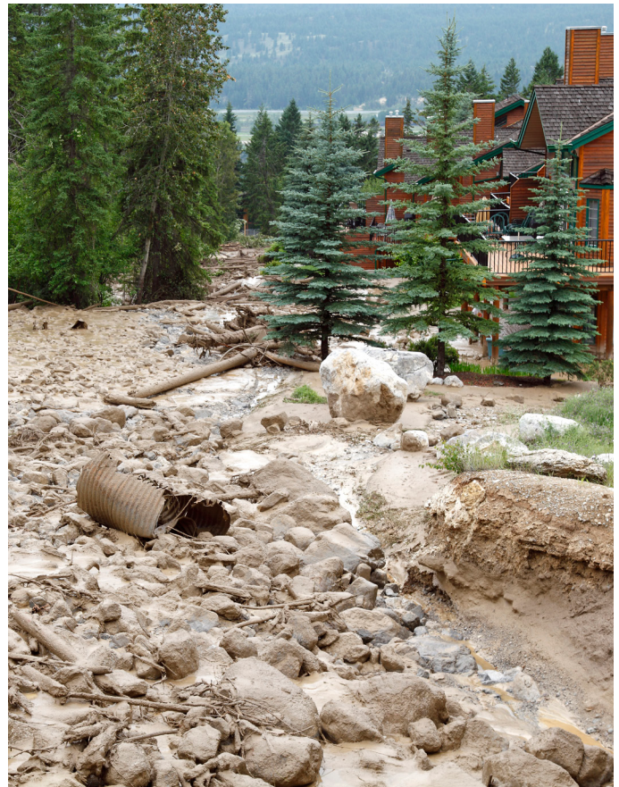
Mud slide with rock, boulders, and debris
