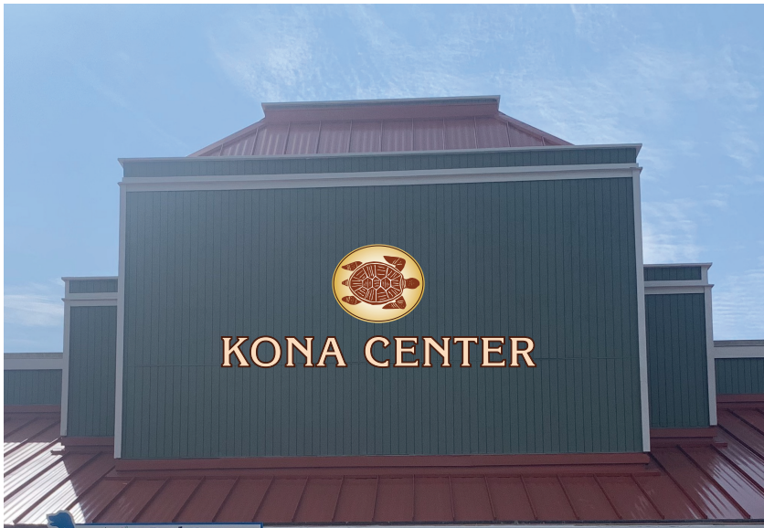
MAIN WALL MARQUIS SIGN
