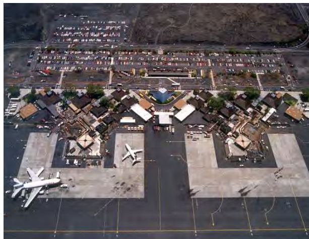
Various Construction Projects, Kona International Airport (1998-2009)
