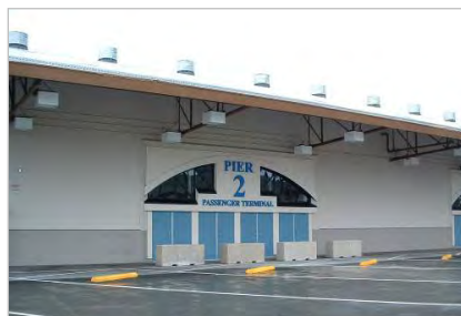
Pier 2 Cruise Terminal, Honolulu Harbor, Oahu (2006)
