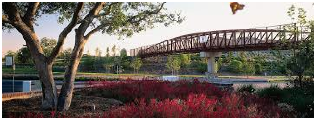
Pedestrian bridge at Ladera Ranch
