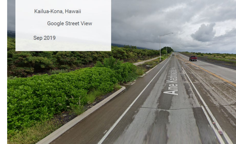
Image along Ane Keohokalole Highway near Manawalea St. Landscaping was installed at curb cuts to filter road runoff. Further down, there is an inlet to a drywell, which is a common method of stormwater infiltration on this island.
