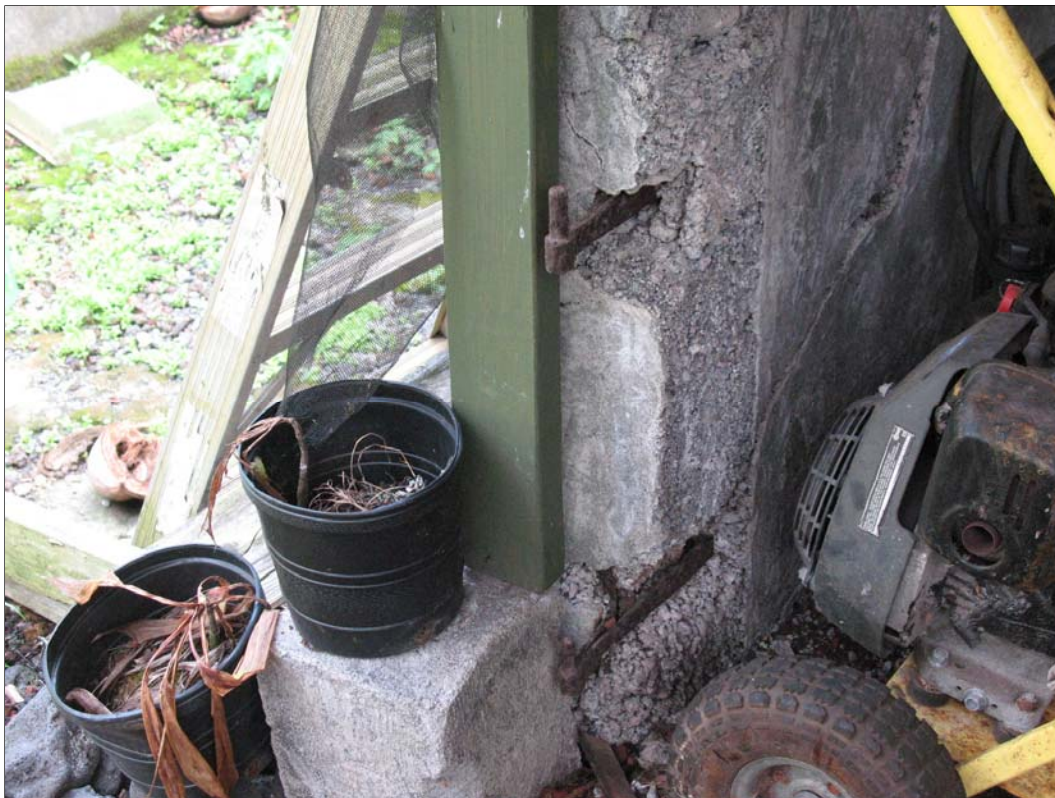
Figure 160. SIHP Site 30133 Feature A, remnant metal pin hinges in easternmost compartment indicating former presence of a door.
