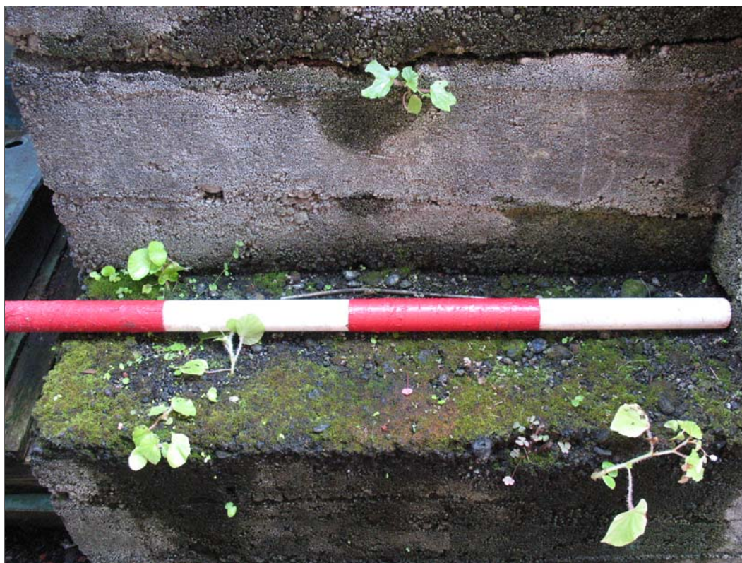
Figure 172. SIHP Site 30134, step area at makai rear corner.
