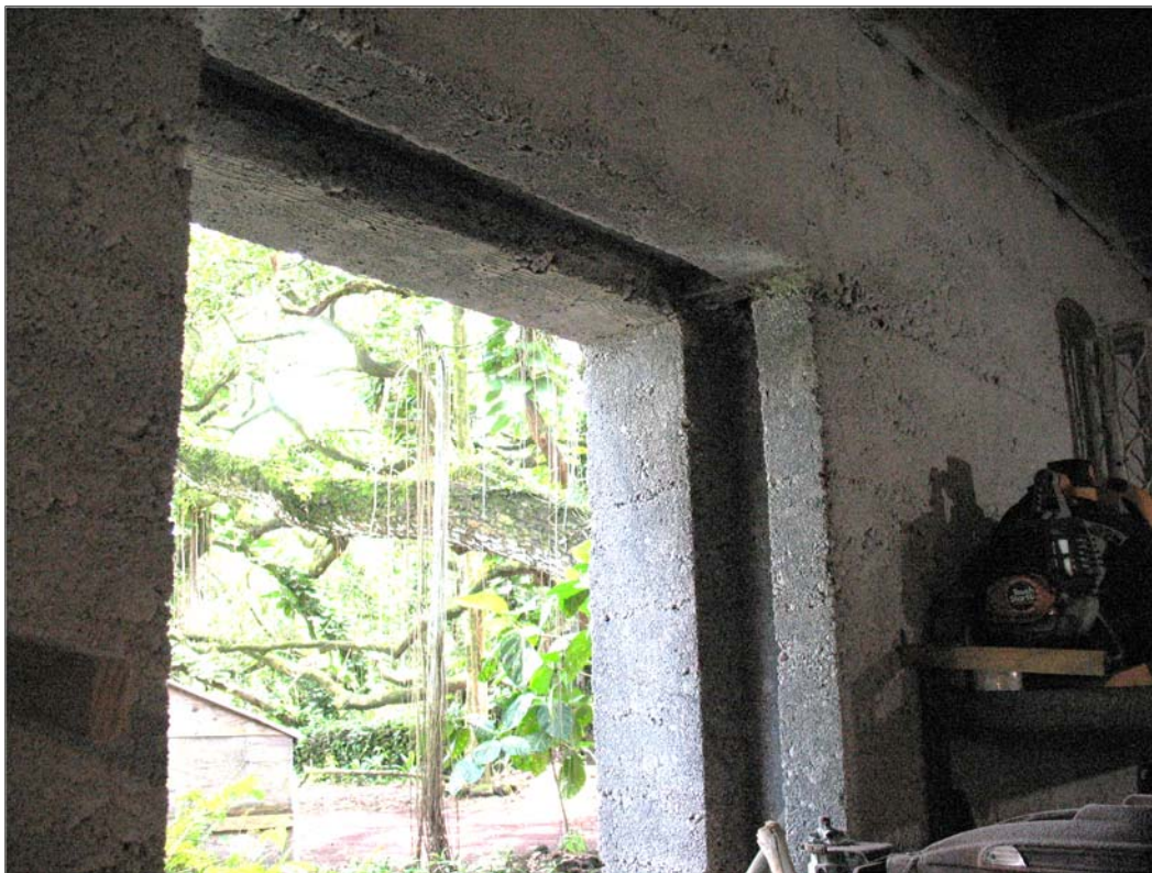
Figure 73. SIHP Site 2511 window opening detail in mill building.
