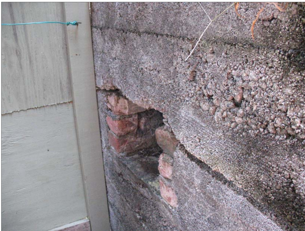
Figure 171. SIHP Site 30134, air vent in back face of structure.
