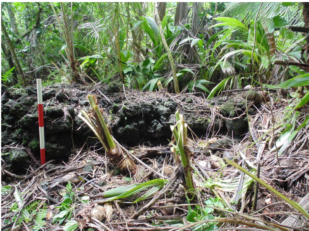
Figure 122. SIHP Site 2516, loosely constructed terrace wall in the makai zone, view to the northwest.
