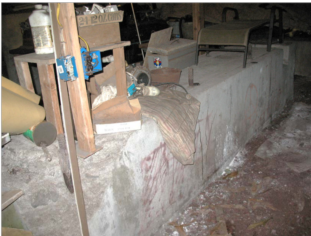
Figure 66. SIHP Site 2511 raised concrete block machinery support in northern third of the mill building.
