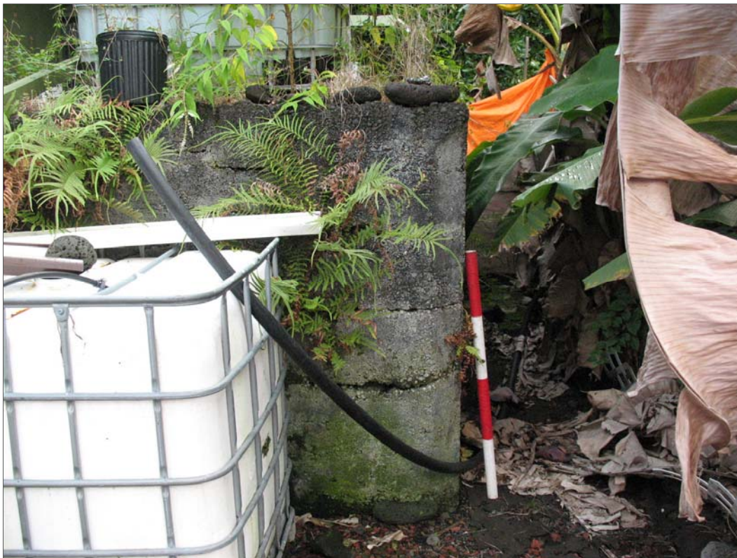
Figure 170. SIHP Site 30134, obscured front of structure, note chamfered corner with lark's tongue finish.
