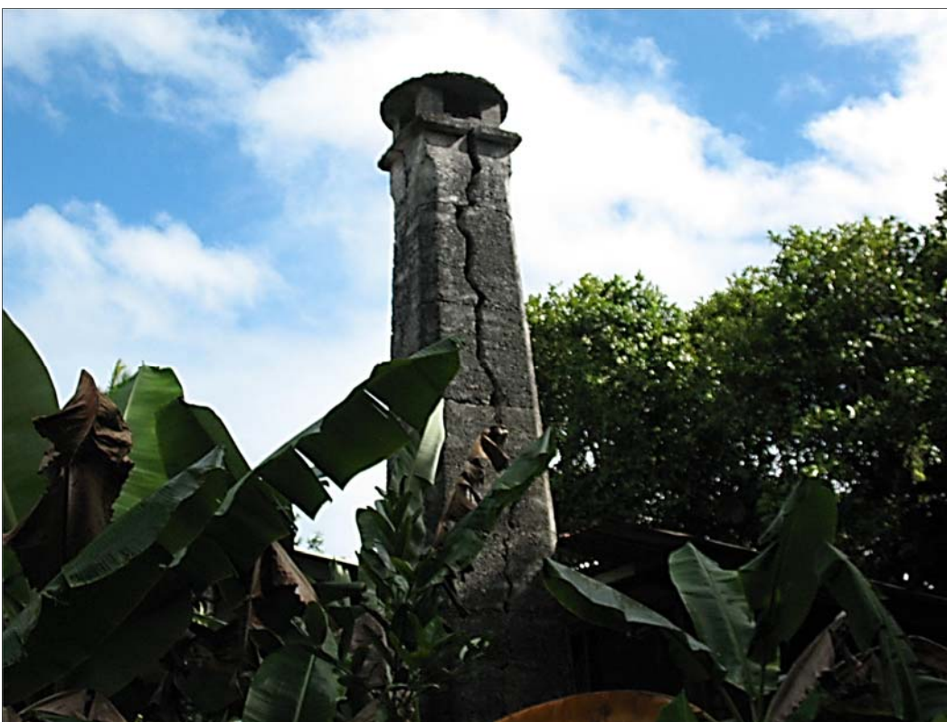
Figure 175. SIHP Site 30134 showing major longitudinal crack in smokestack.
