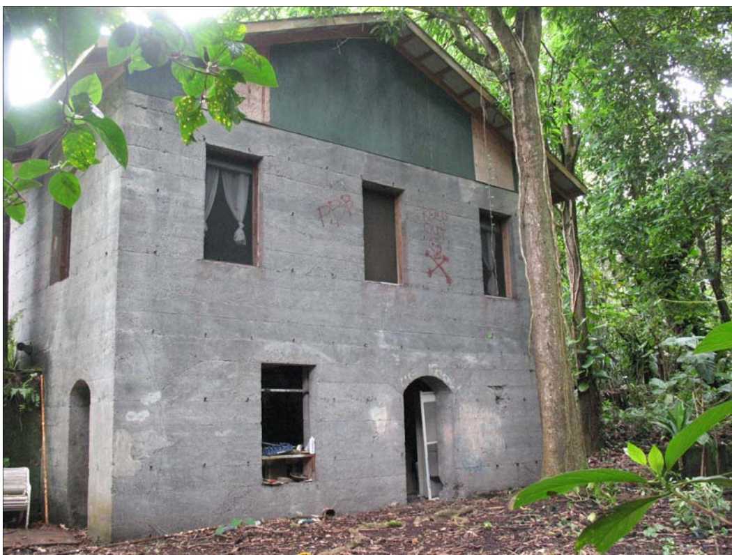
Figure 72. SIHP Site 2511 doorway and four window in northern wall of mill building.
