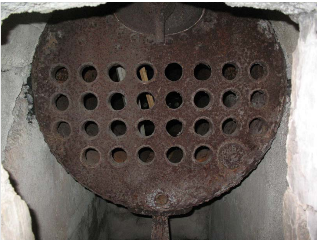
Figure 61. SIHP Site 2511 remaining portion of fire-tube boiler inside mill building.
