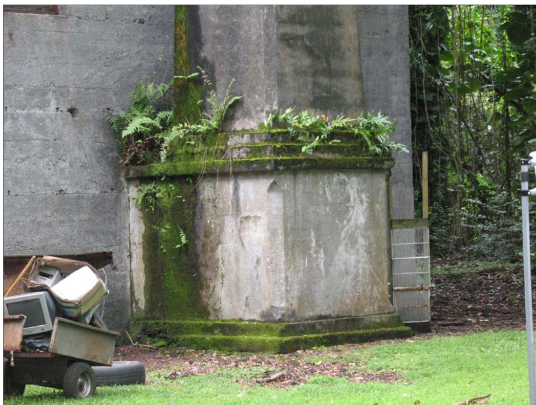
Figure 63. SIHP Site 2511 smokestack base showing chamfer detail.
