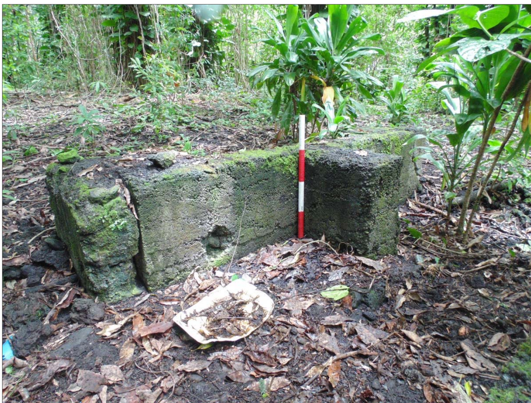
Figure 80. SIHP Site 2511, exterior pier foundation showing shear wall connected mauka piers, view to the southeast.
