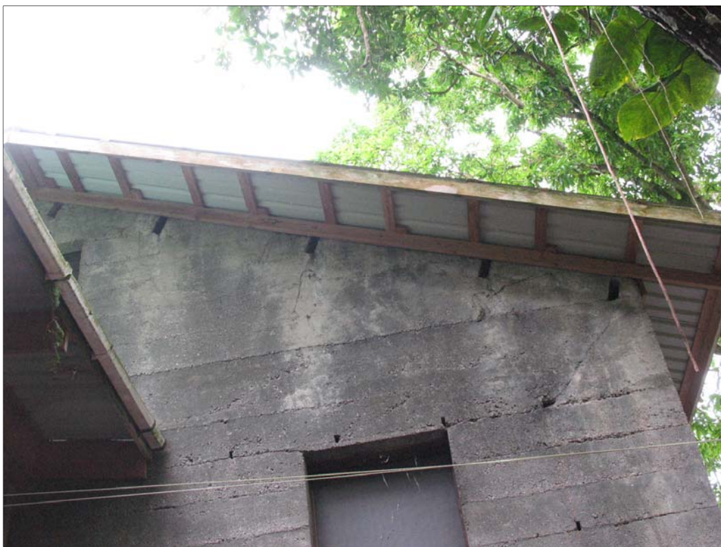
Figure 71. SIHP Site 2511 4 x dimensional lumber voids spaced along top of concrete gable.
