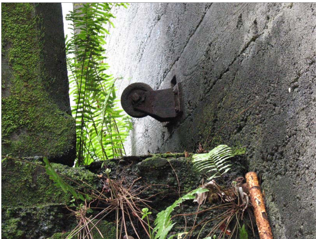
Figure 62. SIHP Site 2511 pulley with cable hole above on eastern exterior wall at smokestack.
