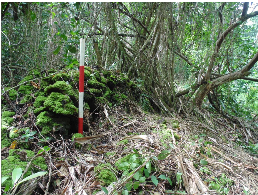
Figure 245. SIHP Site 30146, south end of the wall, view to the northwest.
