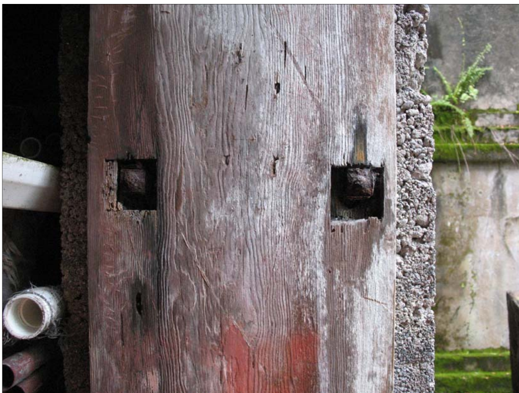
Figure 75. SIHP Site 2511 attached jamb within doorway on ground floor of mill building.
