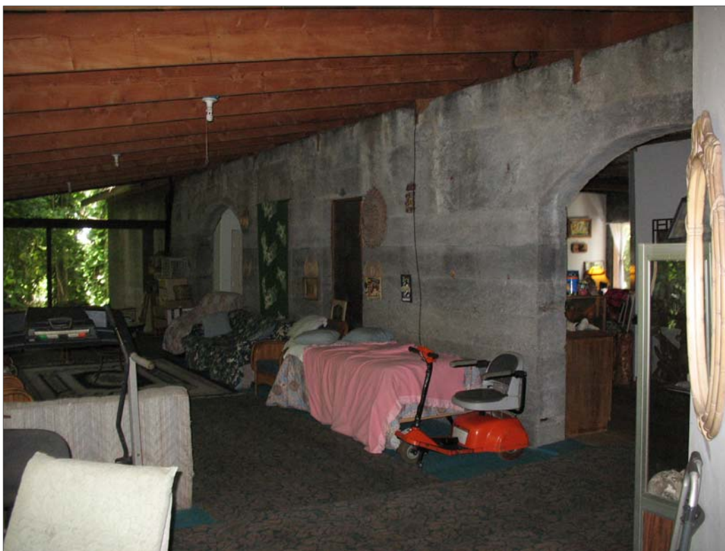
Figure 58. SIHP Site 2511 exterior terrace area as it looks today, enclosed and roofed.
