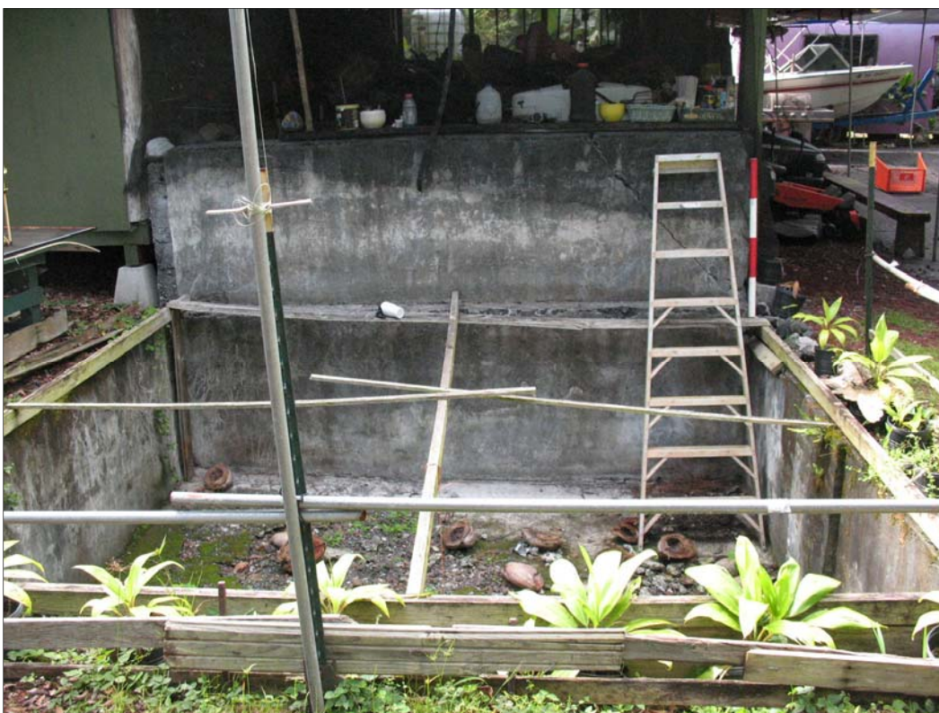
Figure 163. SIHP Site 30133 Feature A, cistern showing connection to easternmost compartment, view to the west.
