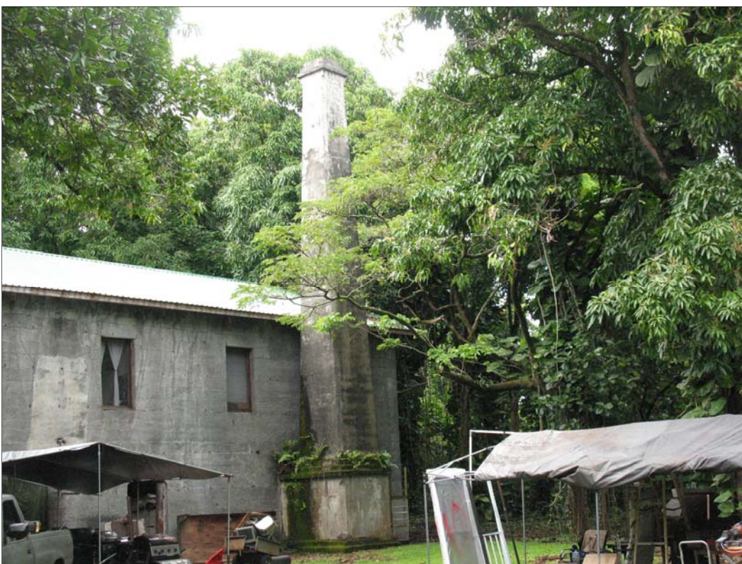
Figure 59. SIHP Site 2511 exterior concrete smokestack, view to the north.
