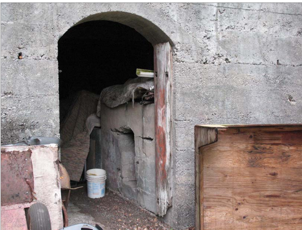
Figure 74. SIHP Site 2511 wooden jamb still present in doorway on ground floor of eastern wall of mill building.
