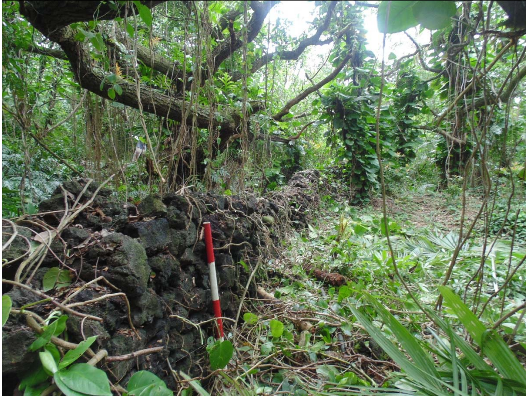
Figure 85. SIHP Site 2515 Feature A, core-filled wall, view to the northeast.
