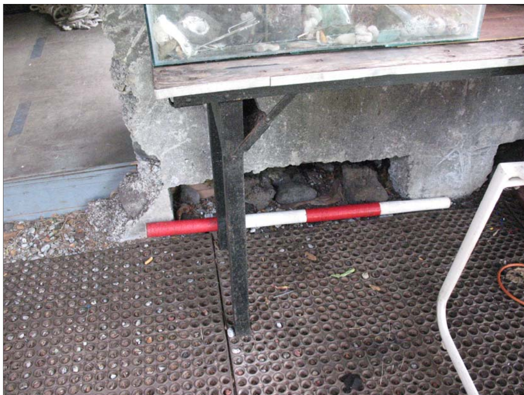
Figure 155. SIHP Site 30133 Feature A, rectangular cleanout in westernmost compartment.
