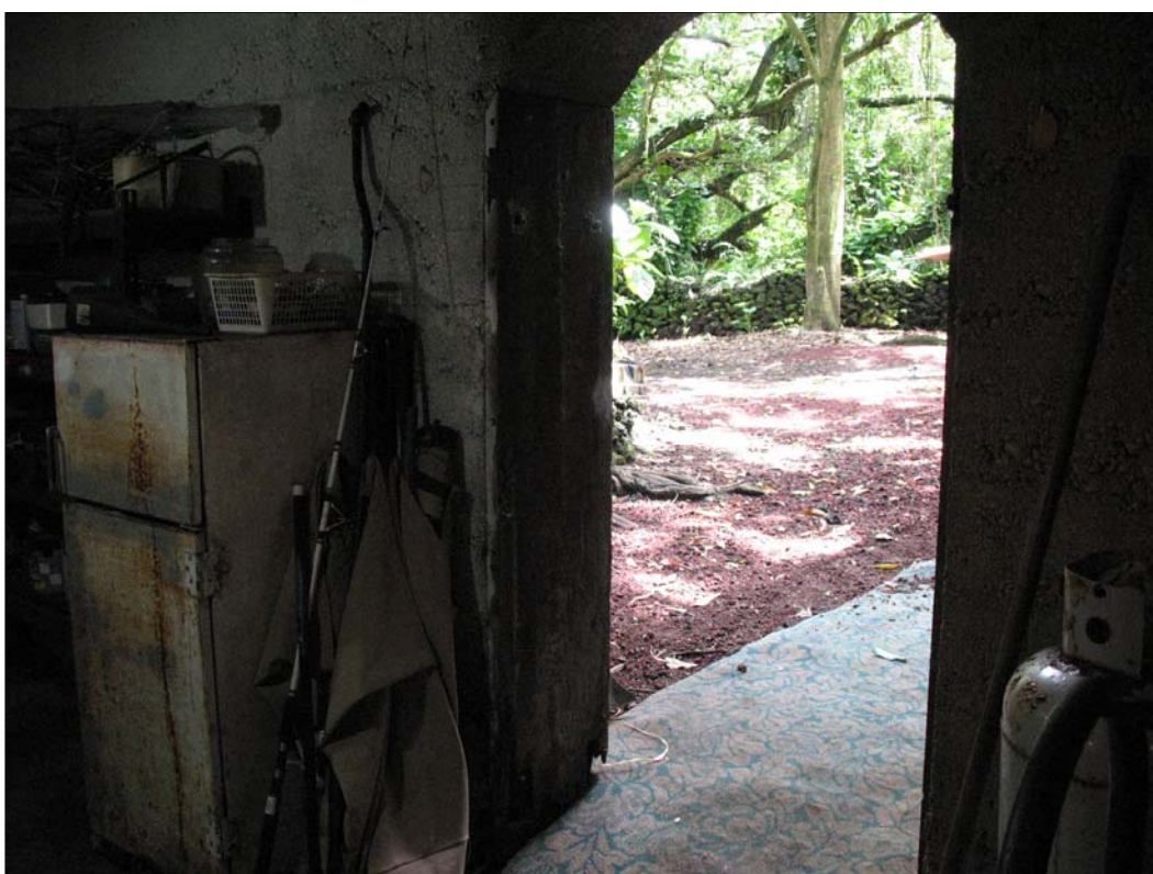
Figure 76. SIHP Site 2511 doorway on ground floor in southern wall of mill building, looking outward.
