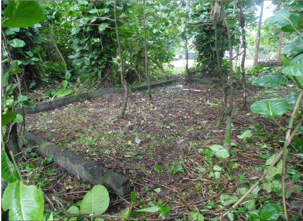
Figure 152. SIHP Site 30132, concrete foundation, view to the southwest.
