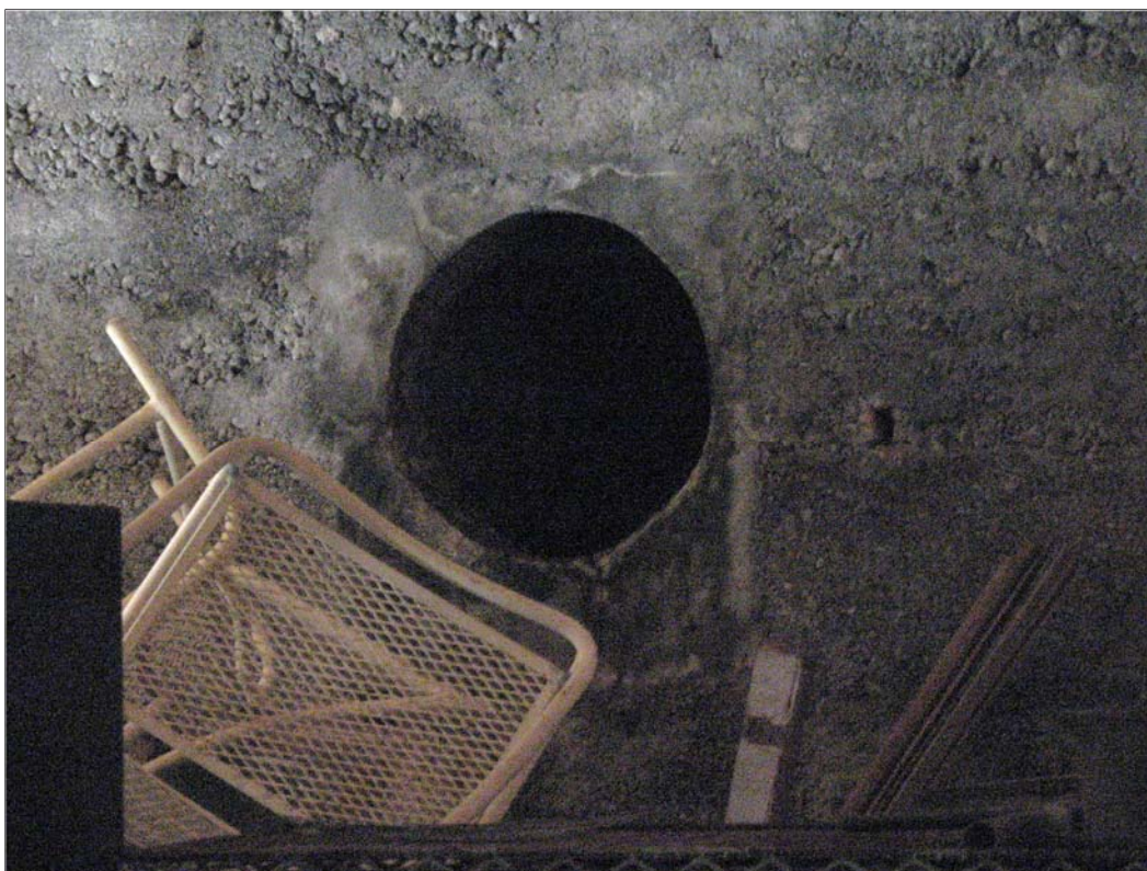
Figure 60. SIHP Site 2511 circular vent hole leading from inside the mill building to the exterior smokestack.
