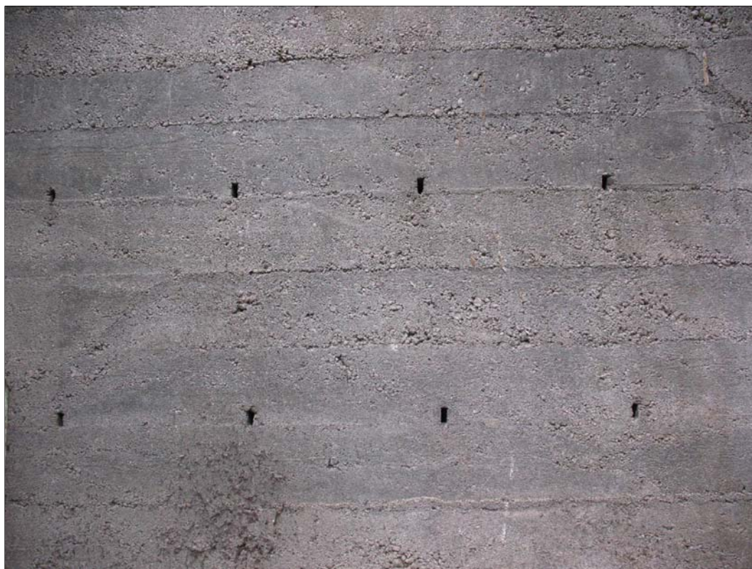
Figure 67. SIHP Site 2511 wooden tie voids and form marks on exterior wall surface.
