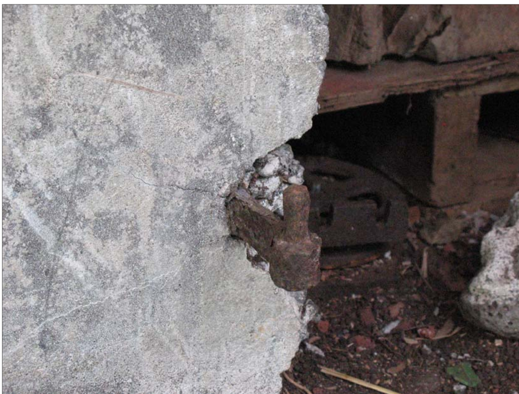
Figure 157. SIHP Site 30133 Feature A, metal pin hinge in concrete next to arched door opening.
