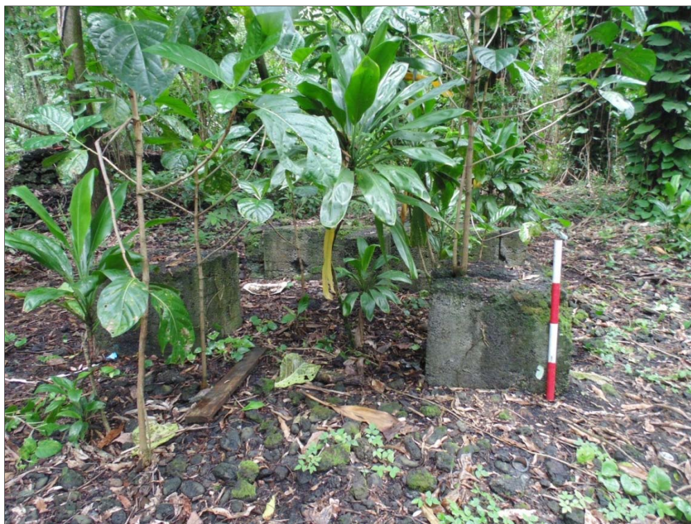
Figure 79. SIHP Site 2511 exterior concrete pier foundation, view to the northwest.
