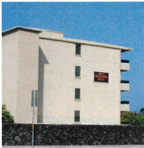
PREVIOUS TENTANTS SIGNAGE View of north facing hotel wall from Kailua Highway
