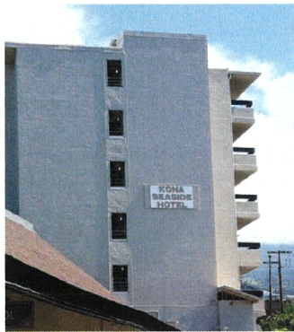
PREVIOUS TENTANTS SIGNAGE View of north facing hotel wall from Ali'i Dr./ Commercial area
