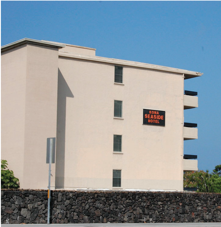
PREVIOUS TENTANTS SIGNAGE View of north facing hotel wall from Kuakini Highway
