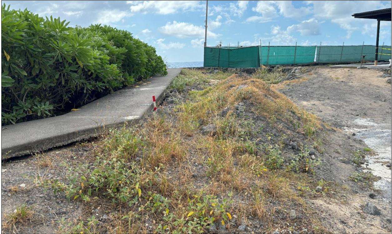
Figure 14. Example of push pile consisting of construction rubble and sand that has resulted from the grading of the development area.
