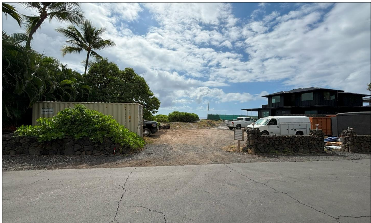
Figure 13. Photo from Kona Bay Drive facing south towards project area illustrating the graded development area.
