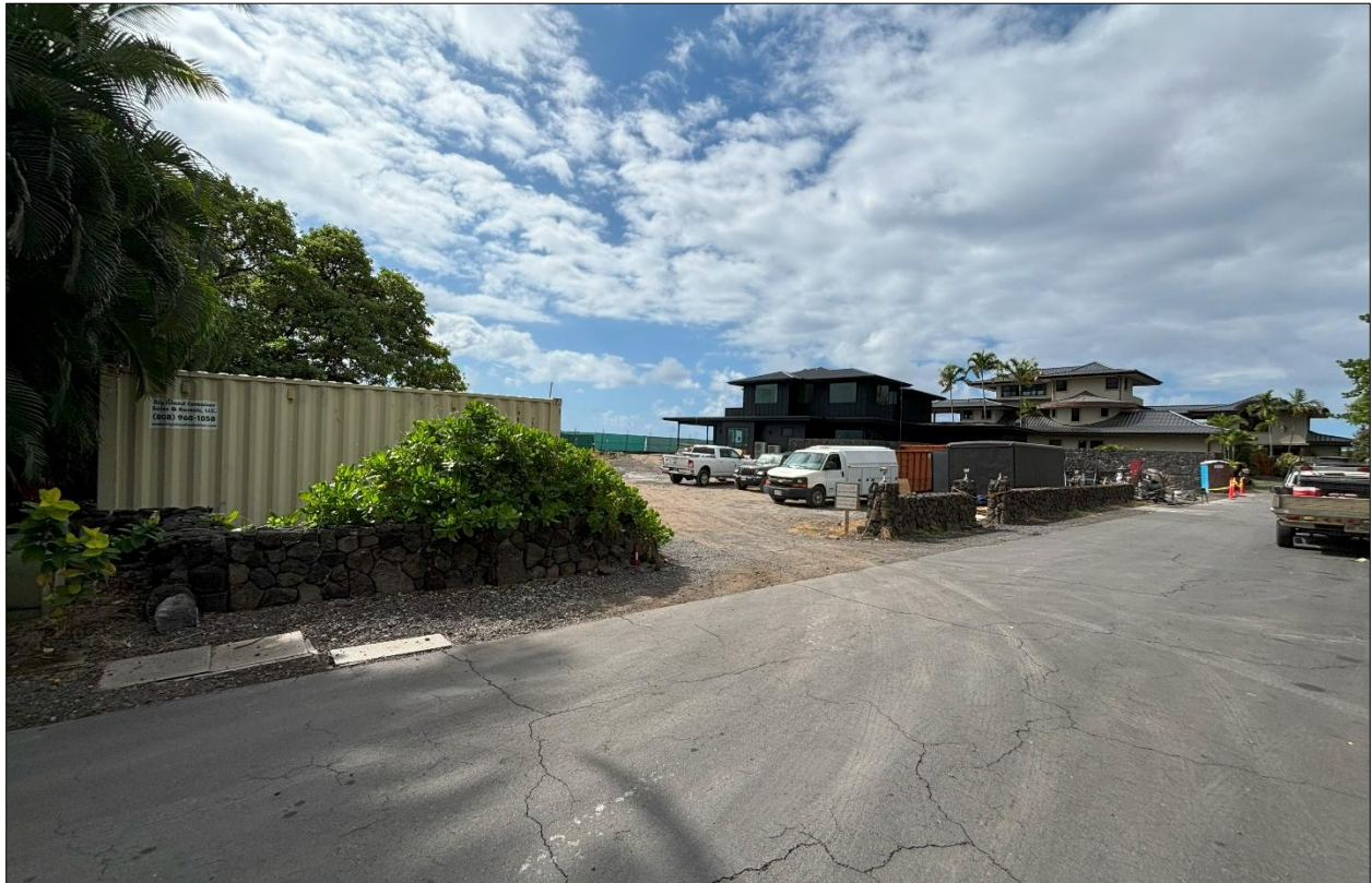
Figure 7. View to the northwest of the project area.
