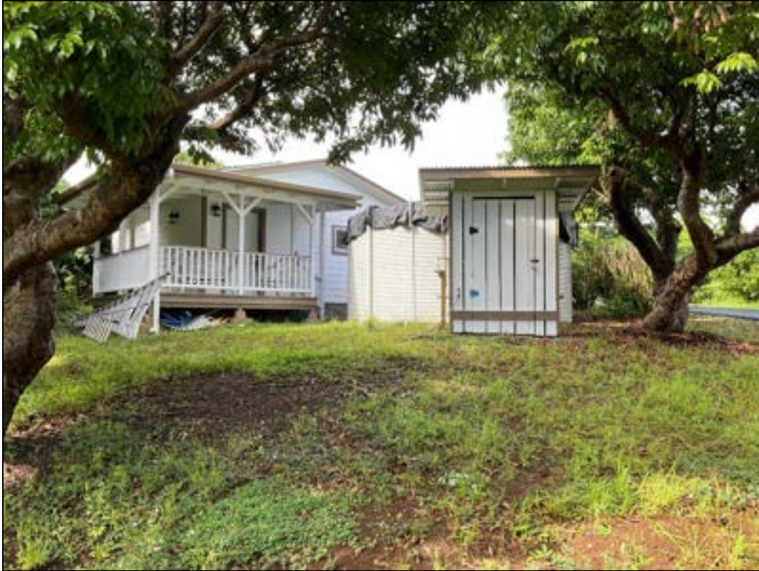
Figure 13. Recently constructed garage, water catchment tank, and shed, view to the west.
