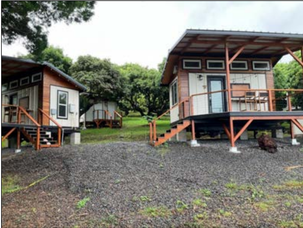
Figure 11. Recently constructed trailered cabins and washroom, view to the south.
