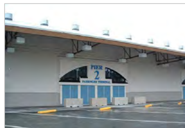
Pier 2 Cruise Terminal, Honolulu Harbor, Oahu (2006)
