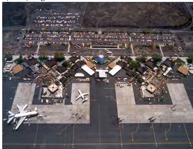
Various Construction Projects, Kona International Airport (1998-2009)
