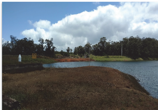
Dam Spillway at the Wahiawa Reservoir
