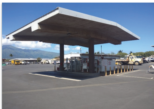
Existing fueling station
