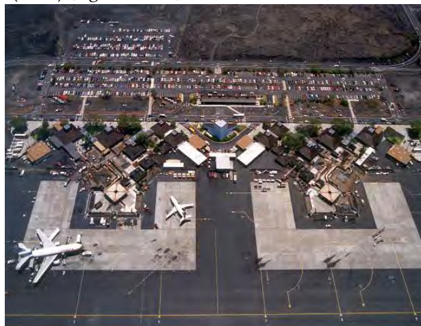
Various Construction Projects, Kona International Airport (1998-2009)
