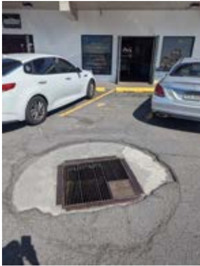
Existing dry well
