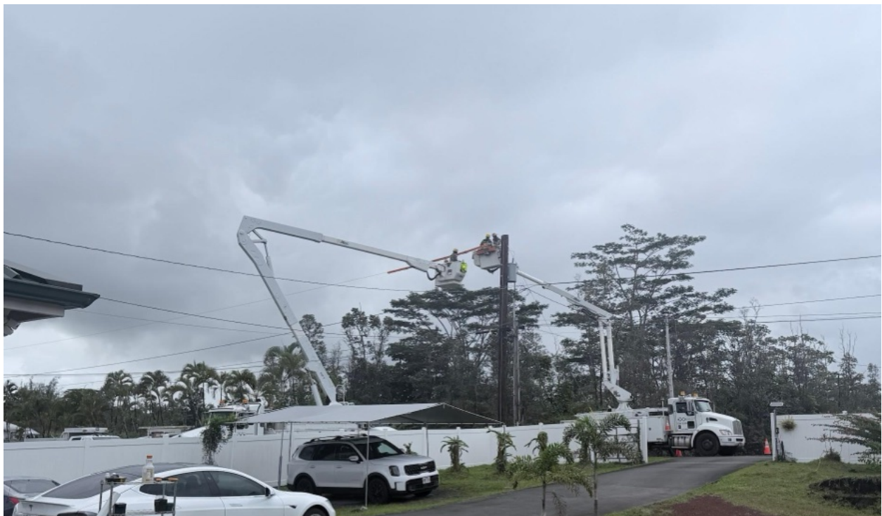
March 3, 2026 - Installing a new utility pole
