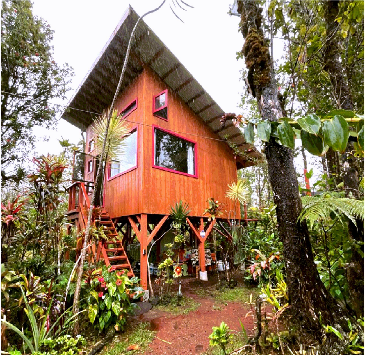
February 9, 2023 Site Inspection
