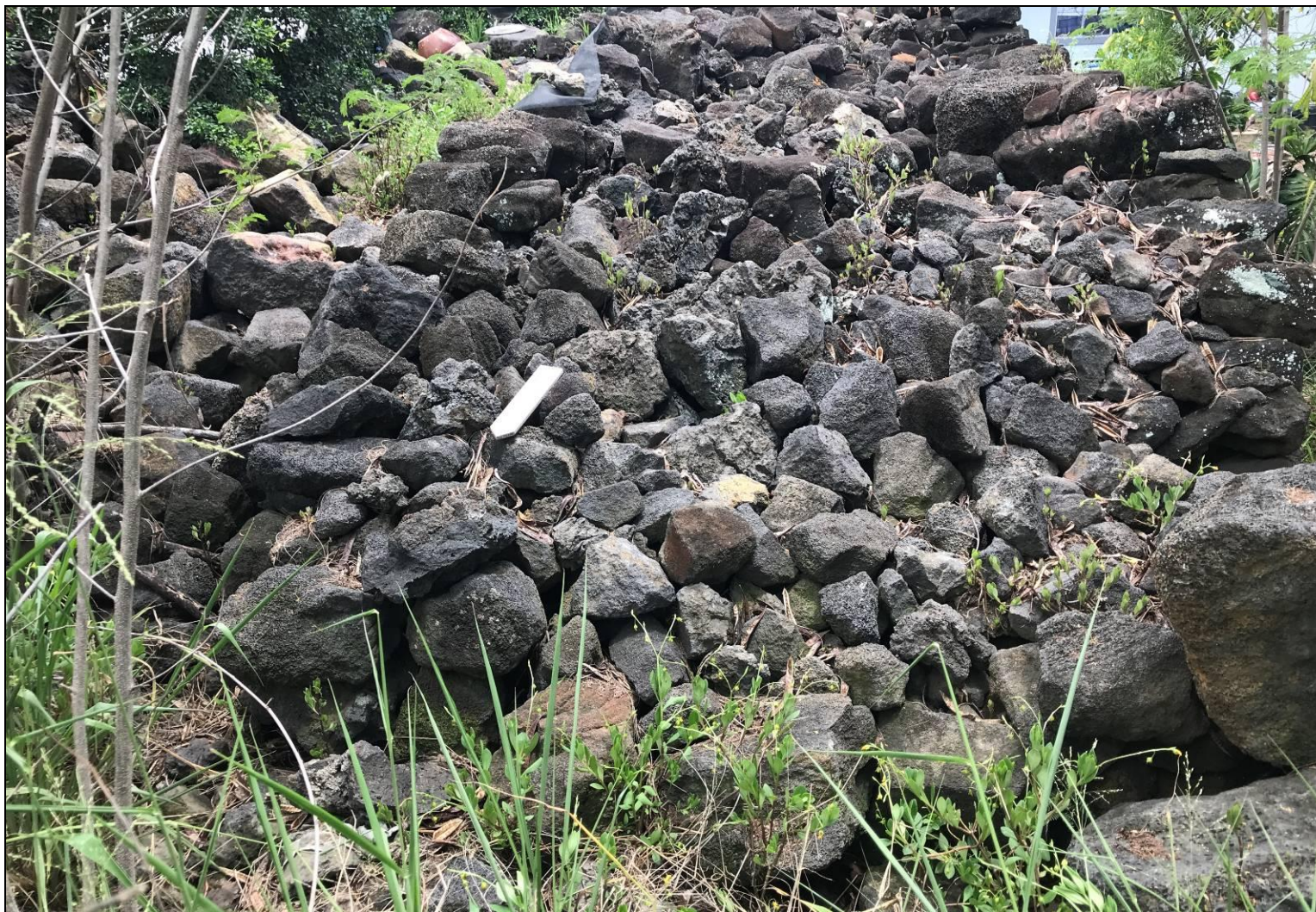
Enclosure 18: Photograph of Stabilized North End of the Southern Segment of Kuakini Wall Site 7267, Looking South (25 cm North Arrow Scale).
