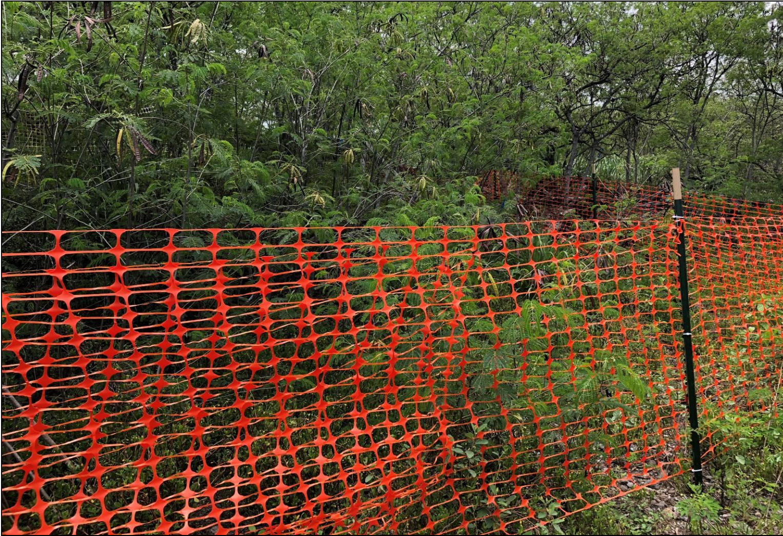
Enclosure 15: Photograph of Site 13673 Construction Buffer Fencing, Looking Southeast.
