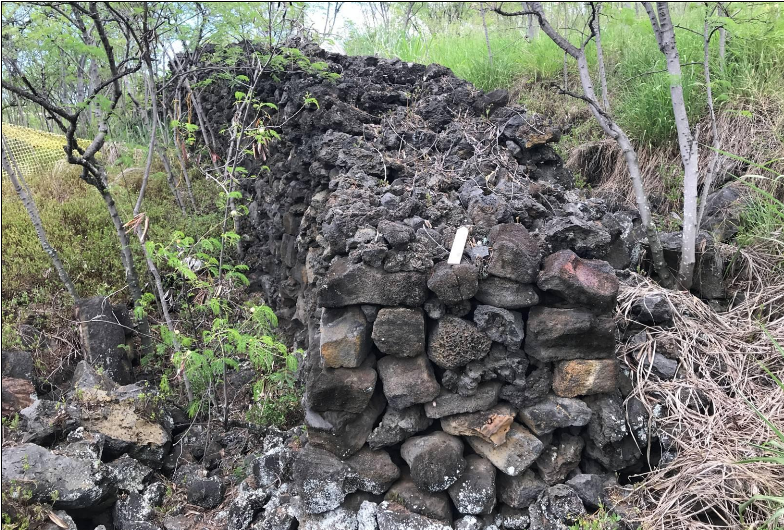
Enclosure 17: Photograph of Stabilized South End of the Northern Segment of Kuakini Wall Site 7267, Looking North (25 cm North Arrow Scale).
