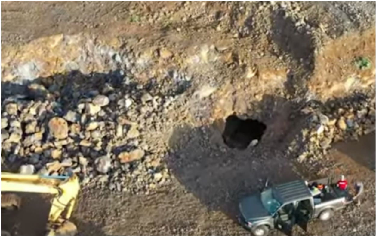
Caption: Aerial photograph showing the surface opening that exposed the lava tube within a disturbed construction zone, compromising the isolation of the cave interior and elevating risk of disturbance, infilling, and environmental exposure.
