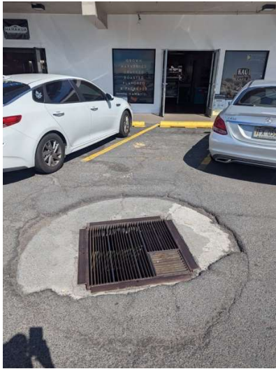
Existing dry well
