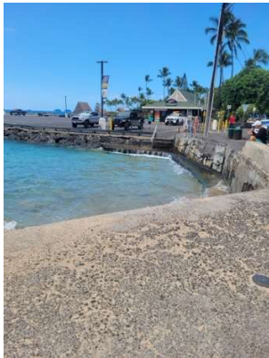
Three steps at Pier
