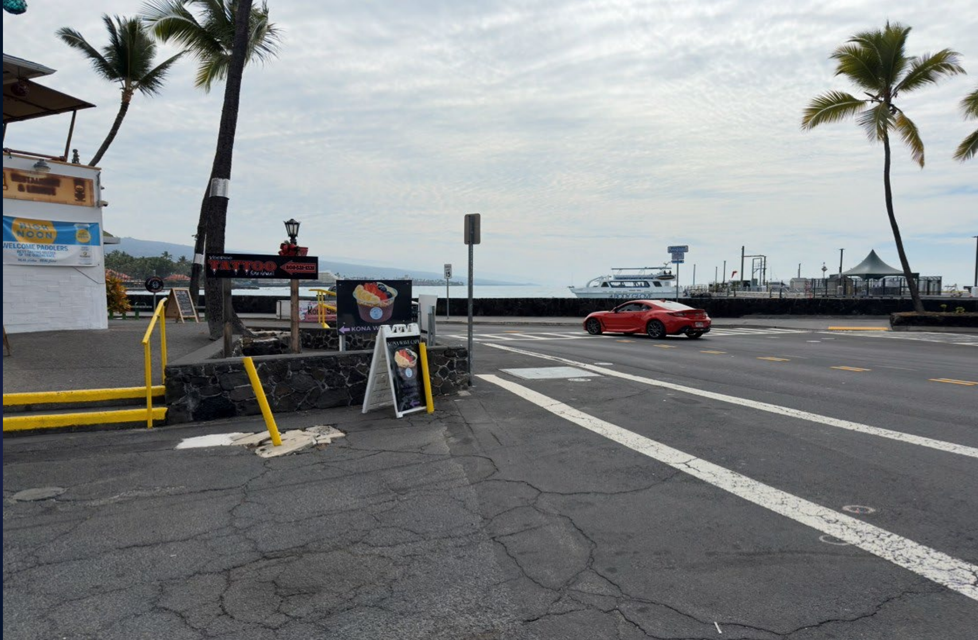
SITE PHOTOS: Southwest
