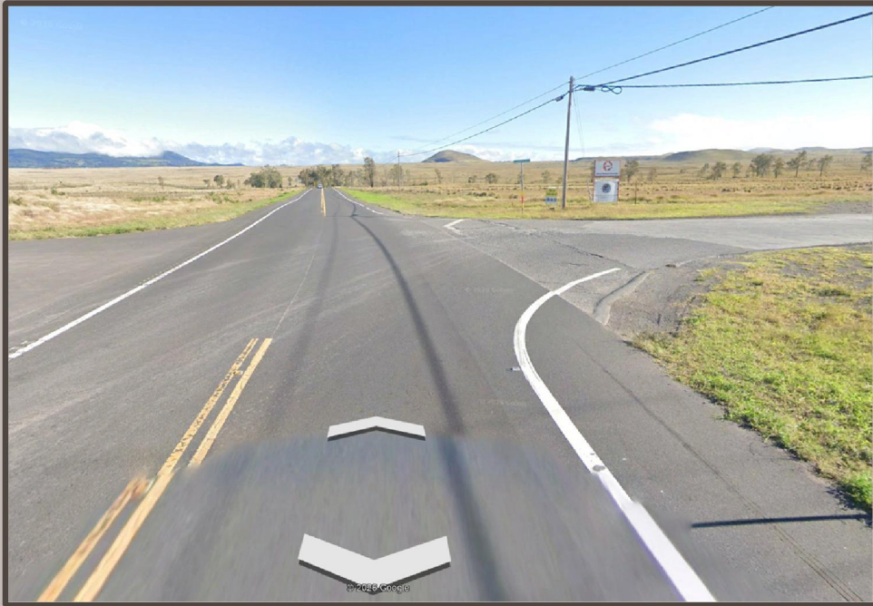
INTERSECTION OF MĀMALAHOA HIGHWAY & QUARRY ACCESS ROAD LOOKING NORTH
