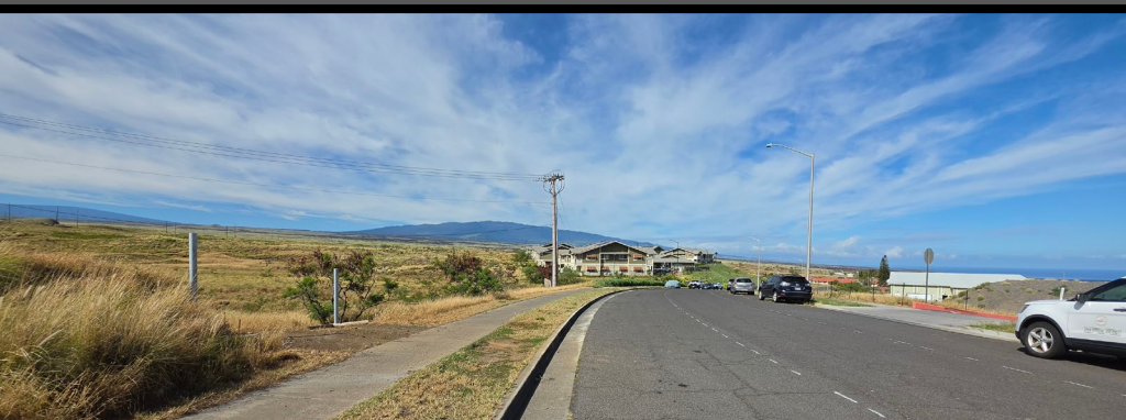
① VIEW OF PUA MELIA STREET FACING SOUTH
