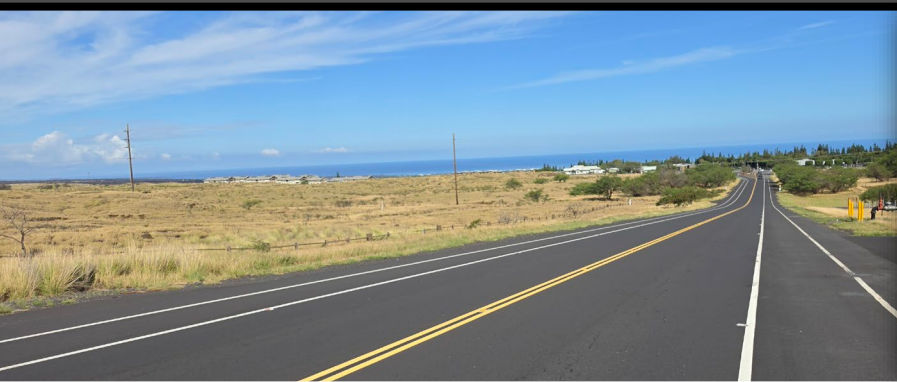
② VIEW OF WAIKŌLOA ROAD FACING MAKAI
