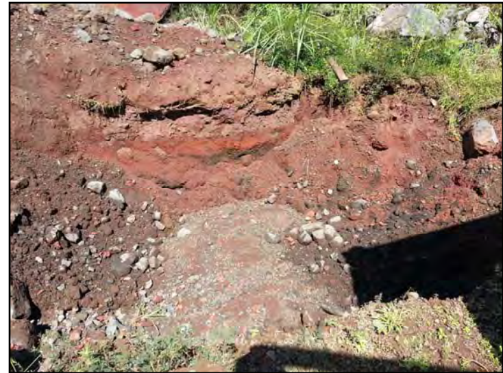
Photograph 4. A view of the catch basin at the northeast end of the subject property (October 30, 2012).
