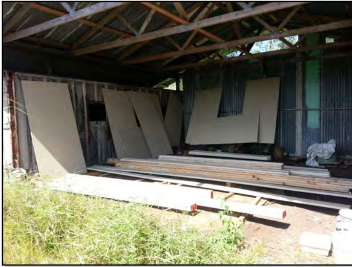
Photograph 17. A view of the shed on the subject property (October 30, 2012).
