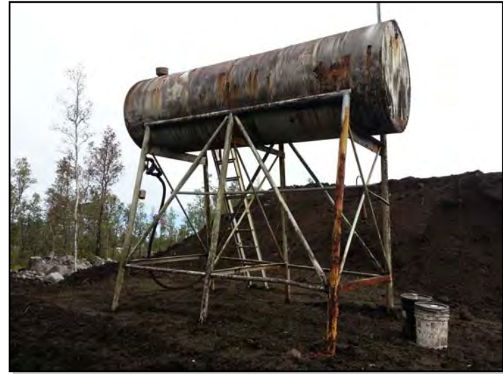
Photograph 50. A view of an old diesel AST on the adjoining property to the north of the west end of the subject property, TMK 1-5-007:007 (October 30, 2012).
