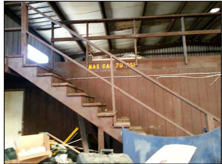
Photograph 16. A view of the stairwell within the warehouse of the subject property (October 30, 2012).
