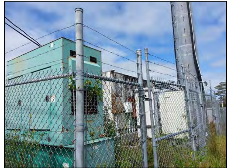
Photograph 24. A view of the fill material to the west of the shed on the subject property (October 30, 2012).
