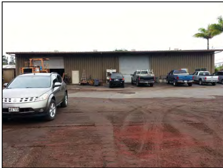
Photograph 5. A view of the warehouse exterior on the subject property (October 30, 2012).
