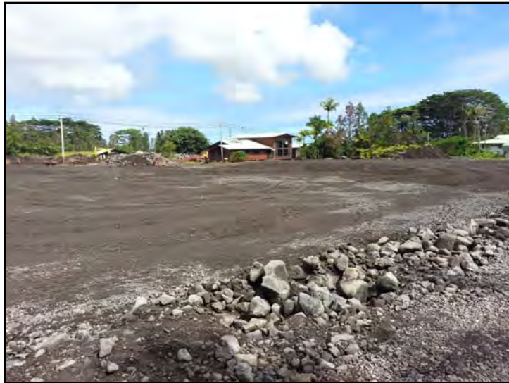
Photograph 3. A view facing northeast from the southwest end of the subject property (October 30, 2012).
