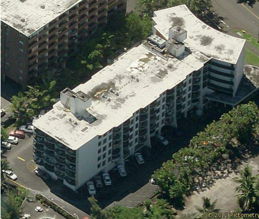
View from North
