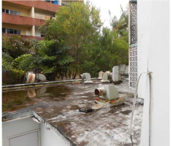
Photo 18: DSCN0480 – Defunct restaurant equipment
