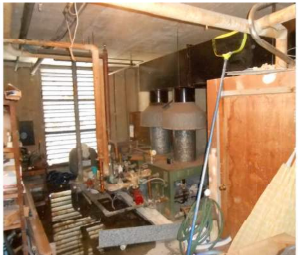
Photo 20: DSCN0461 – Heater/Boiler Room
