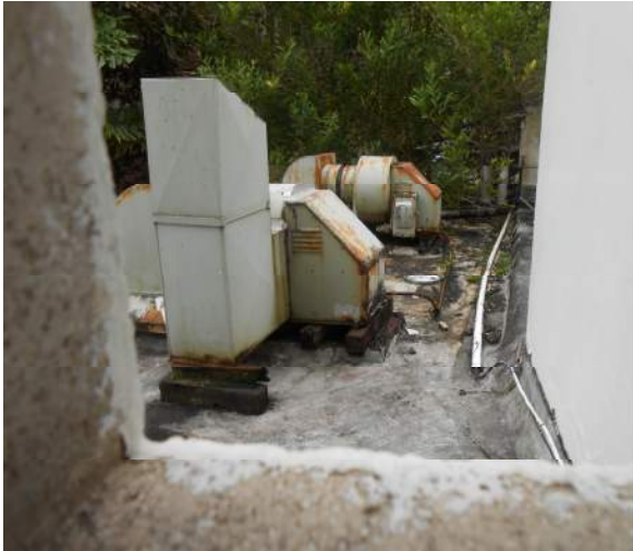
Photo 17: DSCN0479 – Defunct restaurant equipment
