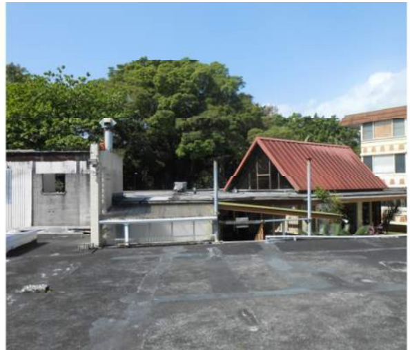
Photo 12: DSCN0434 – Wall and Roof Framing and Restaurant Level
