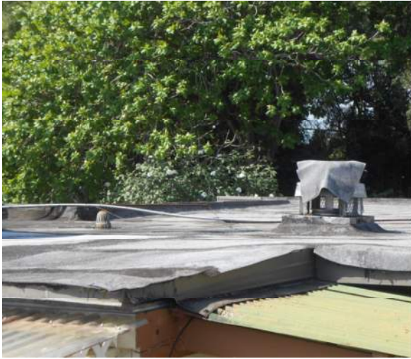
Photo 13: DSCN0431 Roof at Lobby Area
