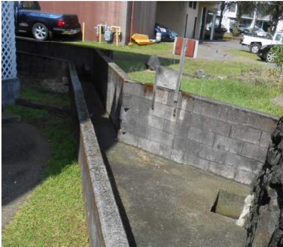
Photo 3: DSCN0443– Concrete Drainage Ditch
