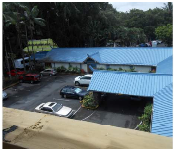
Photo 4: DSCN0519– Aerial view of Parking Lot
