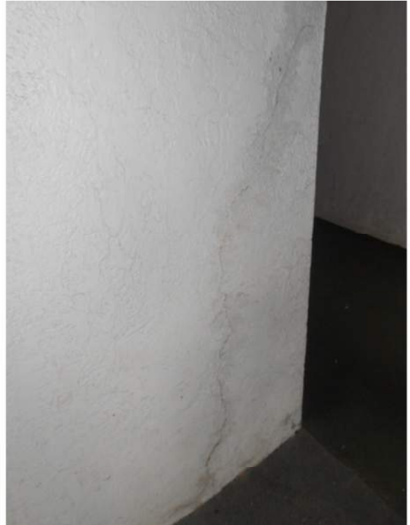
Photo 6: DSCN0490 – Crack with delamination at wall in Kitchen Wing
