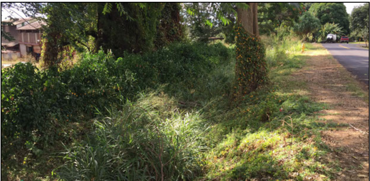
Figure 25. Photo showing the location where the easement in TMK: [3] 9-6-005:036 exits at Ilima Street (frame right); the earthen drainage channel extending from the Huapala Street culvert is beneath the grass to the left of the road; view to southwest
