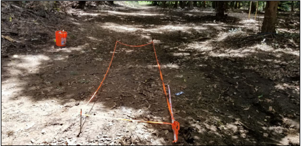
Figure 47. Photo of TE 2 marked out with flagging tape prior to excavation; view to southeast
