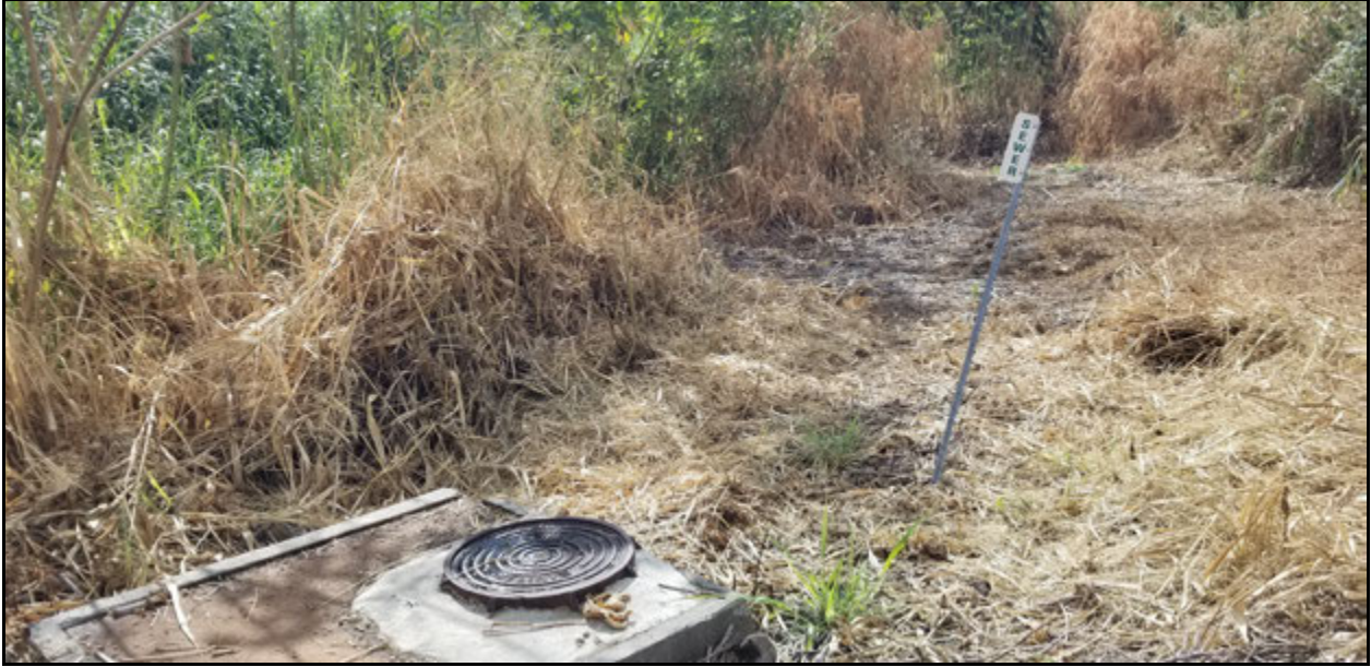
Figure 40. Photo of the sewer manhole located along the existing, maintained sewer easement within TMK: [3] 9-6-002:016; view to southwest
