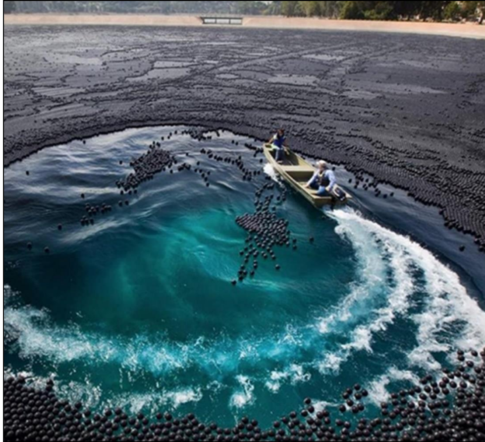
Figure 2.5. Example of Shade Ball Floating Cover in a Lagoon
